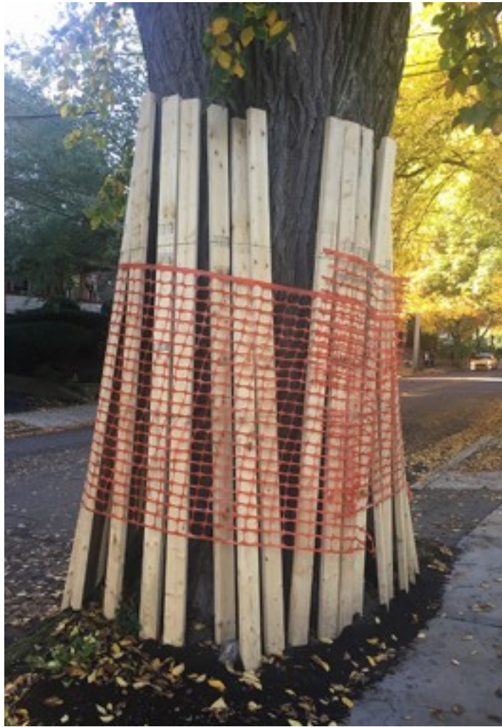
Figure 29 Trunk protection concept for haul road trees falling within potential impact zone (approx. 4') (photo by C.Pepper 2018)
