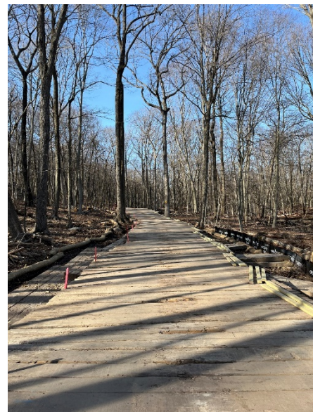
Figure 28 Photo taken mid -March after inventory work showing timber mat haul road
