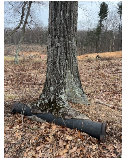
Figure 19 Tree Base Growing Around Original 1920's Irrigation Piping
