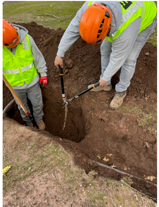
Figure 91 Workers Clean Cutting Roots in Trench
