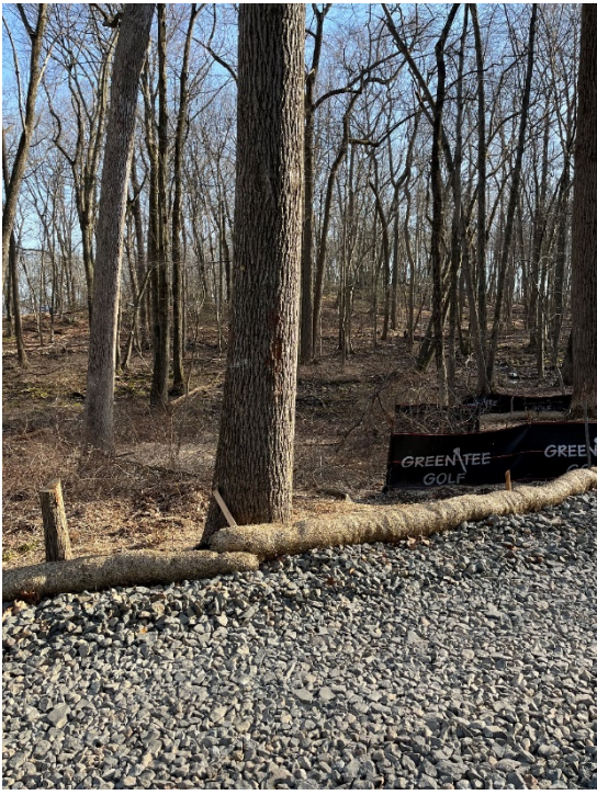
Figure 31 Exposed tree trunk needing protection on exposed on current haul road
