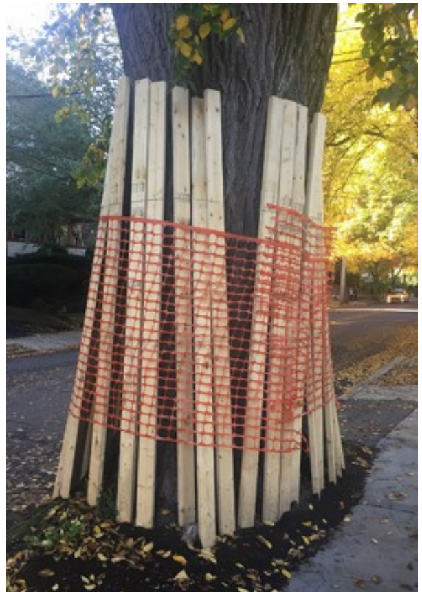
Figure 89 Example of Trunk Protection to Prevent Damage in Construction Zones
