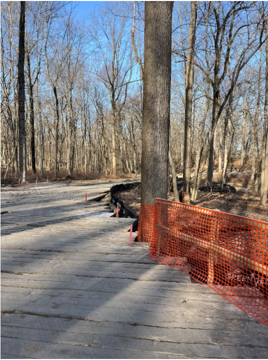
Figure 30 Tree trunk needing protection on current haul road
