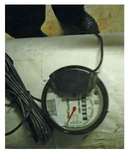
Submeter installed at Central Campus chilled water plant
