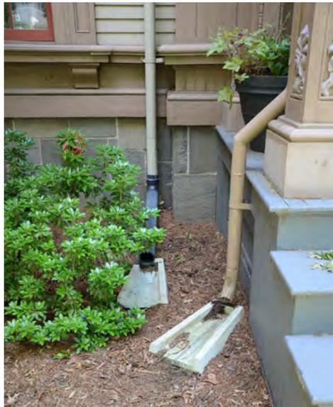
Stormwater from downspouts may also be stored in cisterns for reuse. The cistern behind the Washington, DC, Engine No. 3 fire house, for example, holds rainwater that has been diverted from the buildings' downspouts. The rainwater supplements the potable water required to wash the fire trucks.
