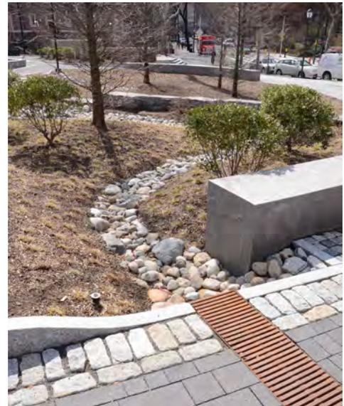
This rain garden and swale collects and stores stormwater from downspouts and a parking lot at the Casey Trees facility in Washington, DC. Hydrophilic trees and native grasses help to soak up and transpire stormwater that would otherwise flow into the area's combined sewer system.
