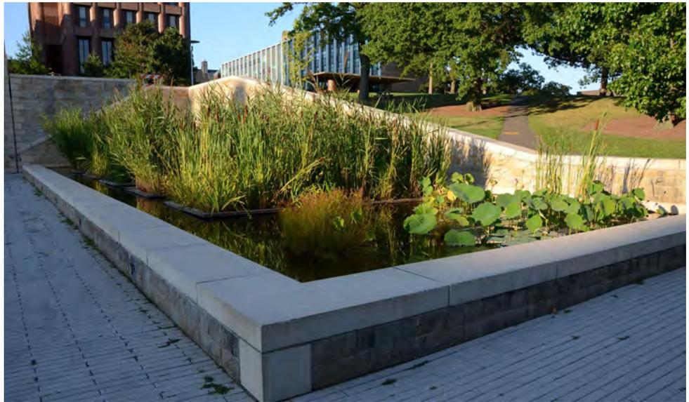
Constructed wetlands may filter stormwater as well as wastewater. This subsurface constructed wetland in the courtyard of the Sidwell Friends School in Washington, DC, utilizes soil and deep-rooted vegetation to filter and recycle wastewater from the buildings' septic system.
