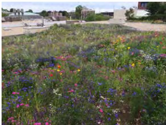
Wright Laboratory was built in 1996 and includes a green roof. More recently, in conjunction with 2016 renovation, Yale Facilities added native vegetation to the roof to enhance both the area's biodiversity and stormwater retention capacity. The project used a pollinator mix that included perennial and annual plantings.
