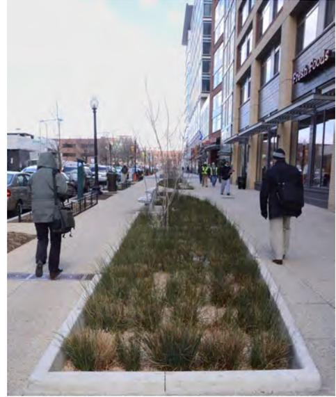
This vegetated bioswale at Kensington High School for the Arts and Performing Arts in North Philadelphia helps to filter runoff from the adjacent parking lot and also receives overflow from nearby improved tree pits. Importantly, bioswales help to capture stormwater and other sediment and debris that would otherwise pollute nearby rivers and streams.
