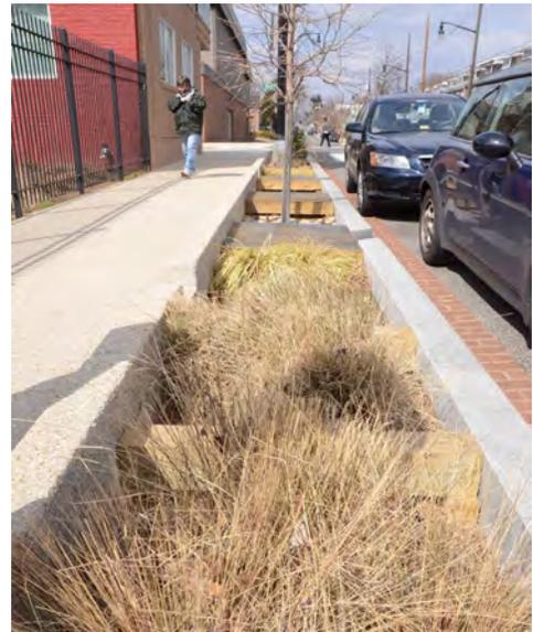
New developments and sites undergoing renovation should be considered for green infrastructure implementation. This bioswale in Washington, DC creates green space and receives stormwater runoff from the right-of-way in a new commercial district.
