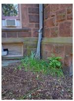
**Downspout 2** Connected. Drains to a small pervious area. Potential for a rain garden of approx. 14 ft. x 8 ft.
