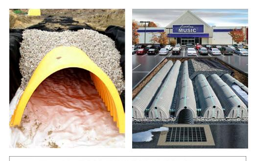
Water infiltrates through the surface and gravel substrate and is conveyed through the perforated pipe into a larger cistern, dry well, or other storage chamber.
