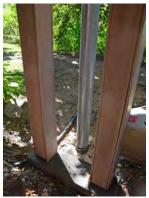
**Downspout 4** Connected. Drains to a pervious area. Potential for a rain garden.
