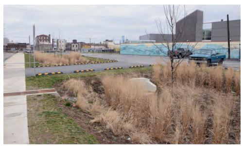
This vegetated bioswale at Kennsington High School for the Arts and Performing Arts in North Philadelphia helps to filter runoff from the adjacent parking lot and also receives overflow from nearby improved tree pits. Importantly, bioswales help to capture stormwater and other sediment and debris that would otherwise pollute nearby rivers and streams.
