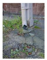
Downspout 3 Disconnected. Drains to a pervious area. Erosion could be reduced with rocks. Potential for rain garden.
