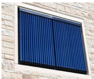
Solar thermal panel creates domestic hot water for immediate use
