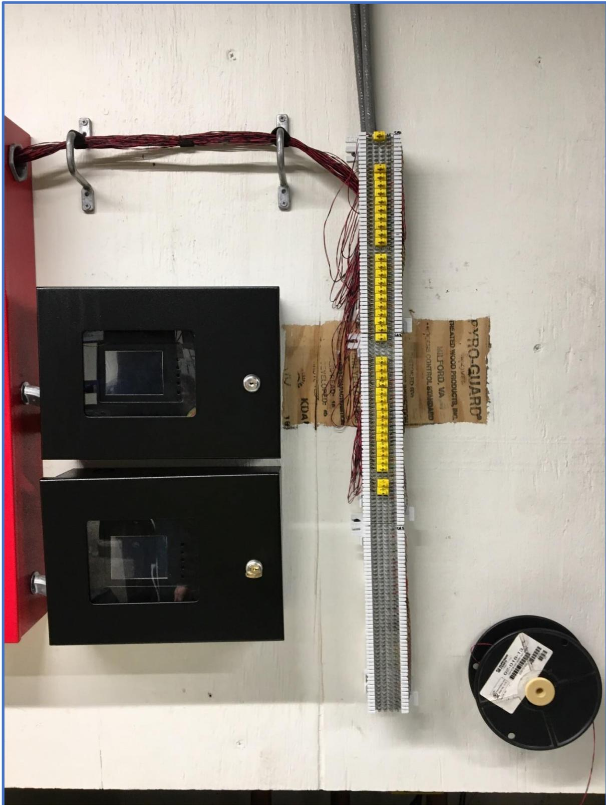
Mass Notification System (MNS) Photo 41 – Copper Pair 66 Block Demarc
