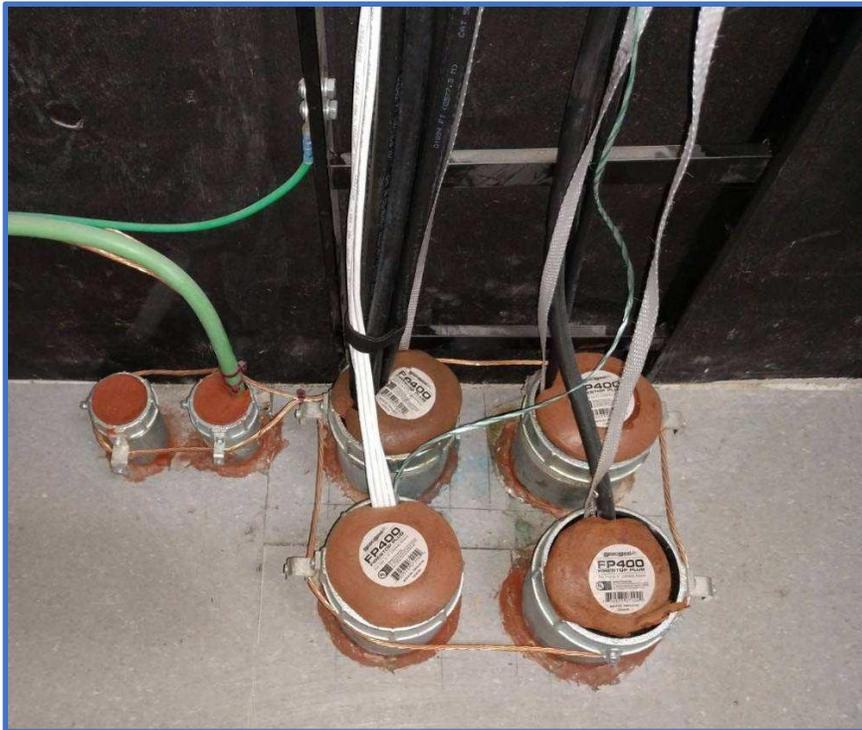
Firestopping Photo 5 – Grounded and Firestopped Conduit Penetration Sleeves
