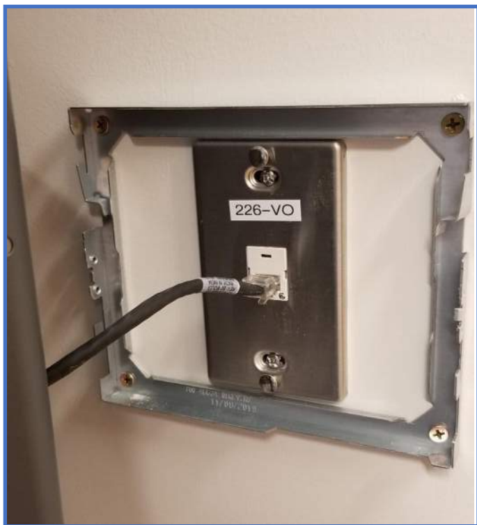
Telecom Outlet Photo 2 – Wall Mounted Telephone Outlet for Cisco VoIP Telephone with Bracket
