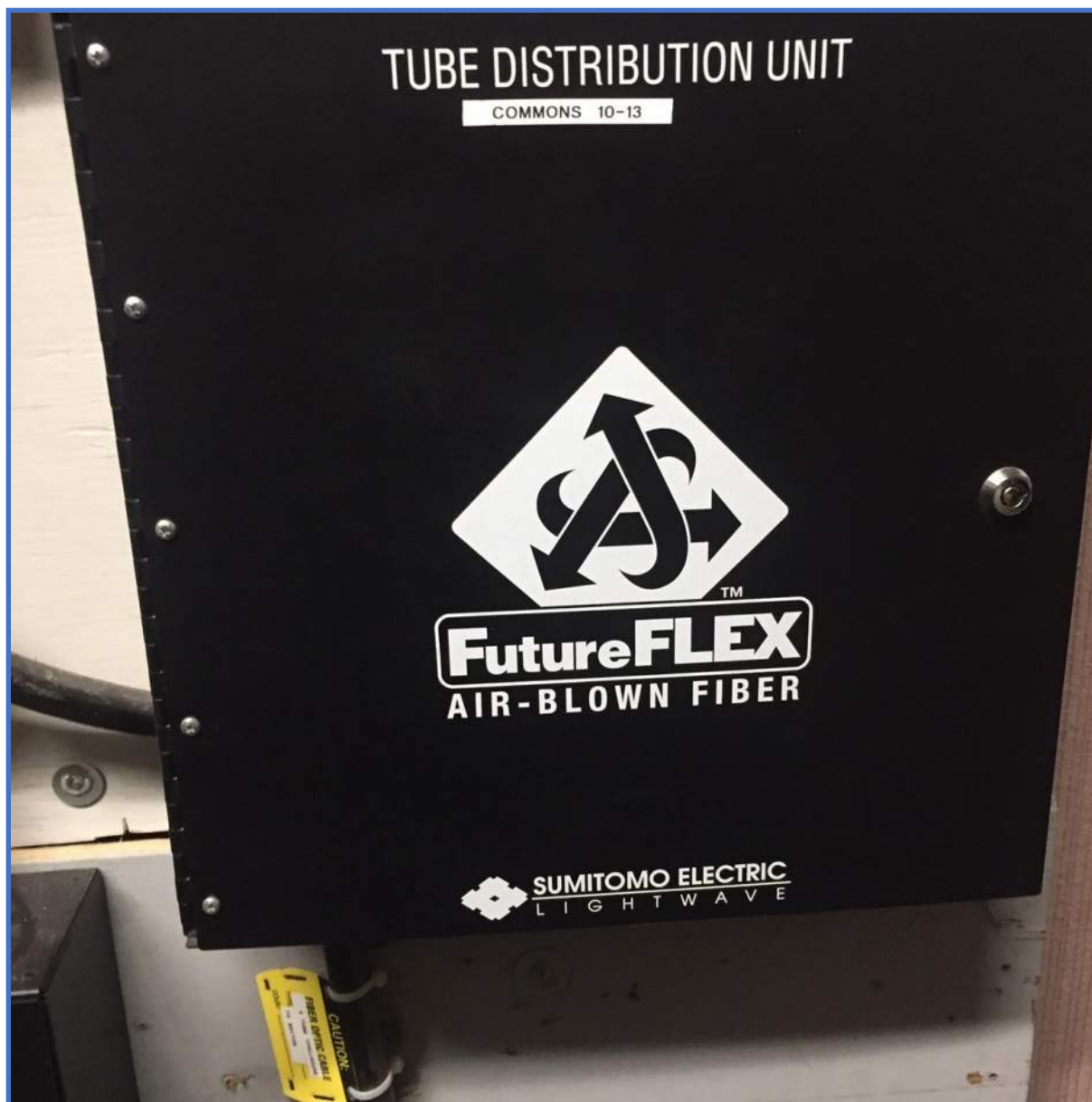
Air Blown Fiber (ABF) Photo 26 – Tube Distribution Unit Wall Field (1)
