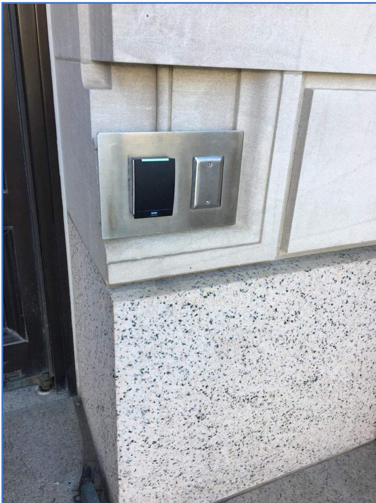
Security System Photo 29 – Device Mounting Integration at Existing Entry
