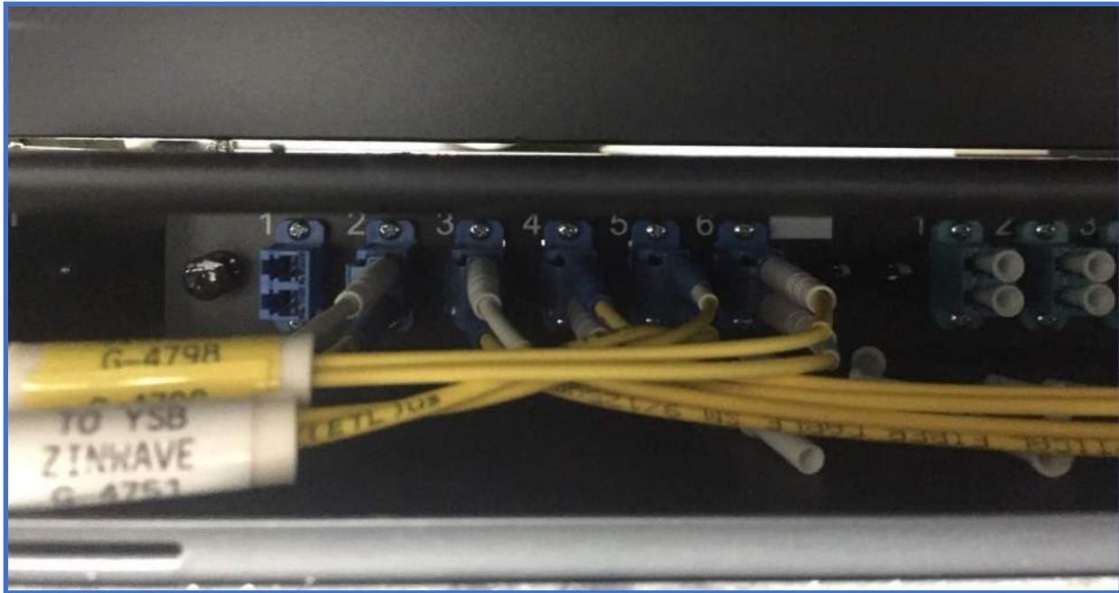
Labeling Photo 24 – Equipment Rack and Optical Fiber Riser Termination Cabinet
