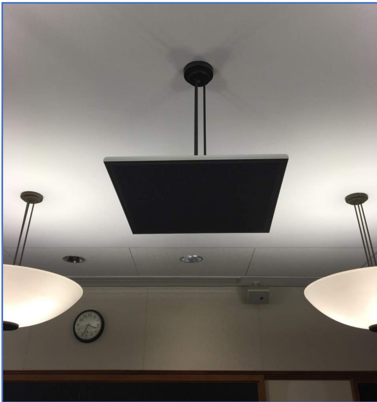
Ceiling Array Microphone Photo 7 – Ceiling Array Microphone with Custom Pendant Mount (Shure MXA910 Series)
