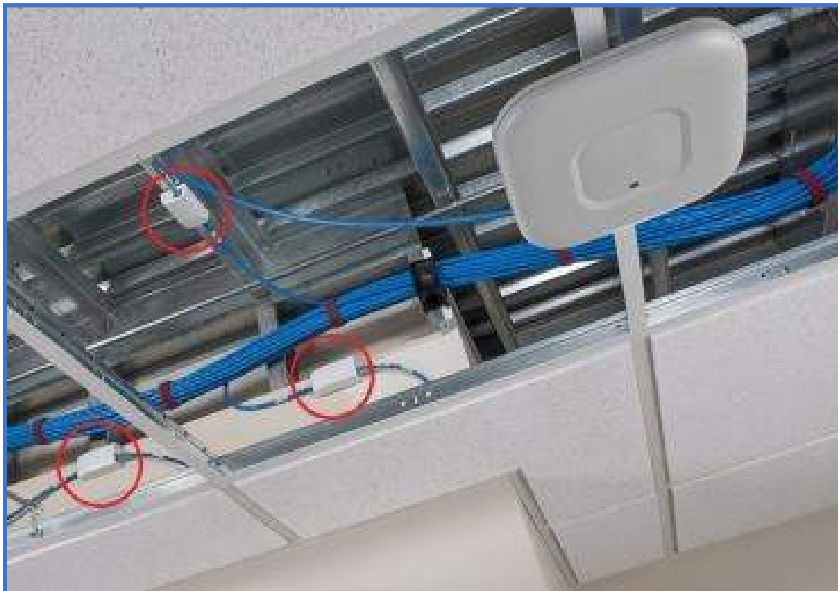
Wi-Fi Photo 37 – Wireless Access Point Biscuit Style Telecom Outlet Supported From Building Structure
