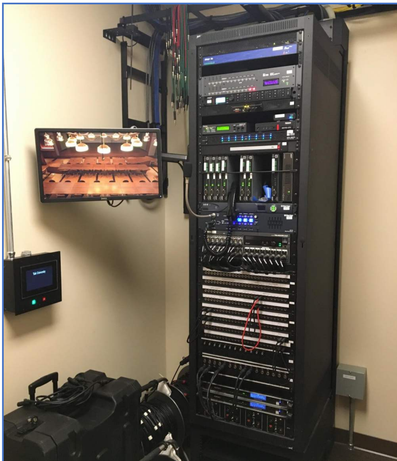
Audiovisual Cabinet Photo 14 – Wall Mounted Rotating Wall Cabinet Installation
