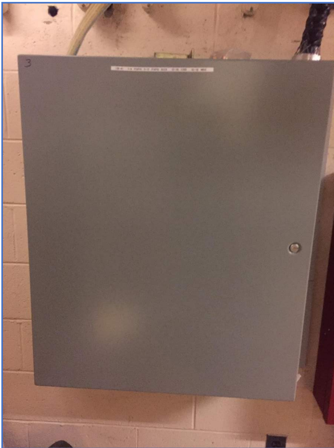
Air Blown Fiber (ABF) Photo 27 – Tube Distribution Unit Wall Field (2)
