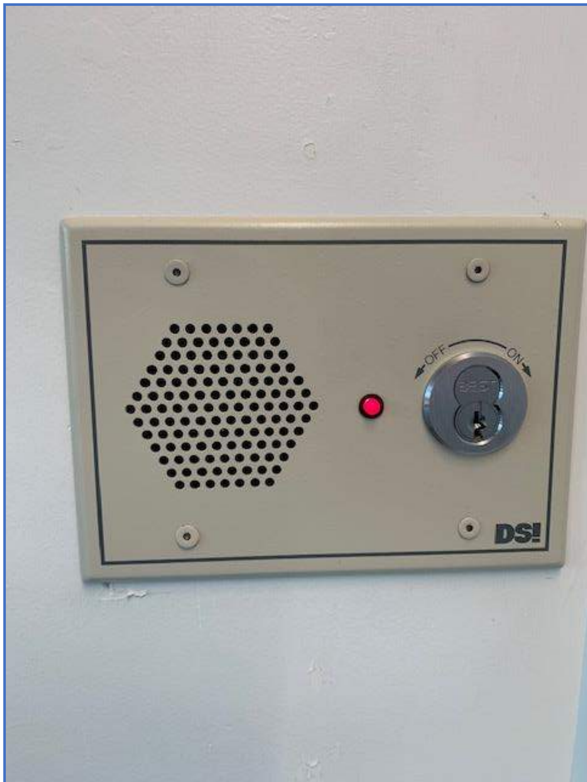
Security System Photo 13 – Door Management Alarm Panel with Key Override
