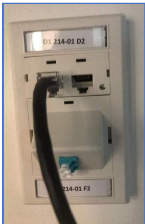
Telecom Outlet Photo 4 – Two (2) Category 6/Two (2) Strand 50 Micron OM4 with LC Duplex Connector for Fiber to the Desktop (FTTD) outlet
