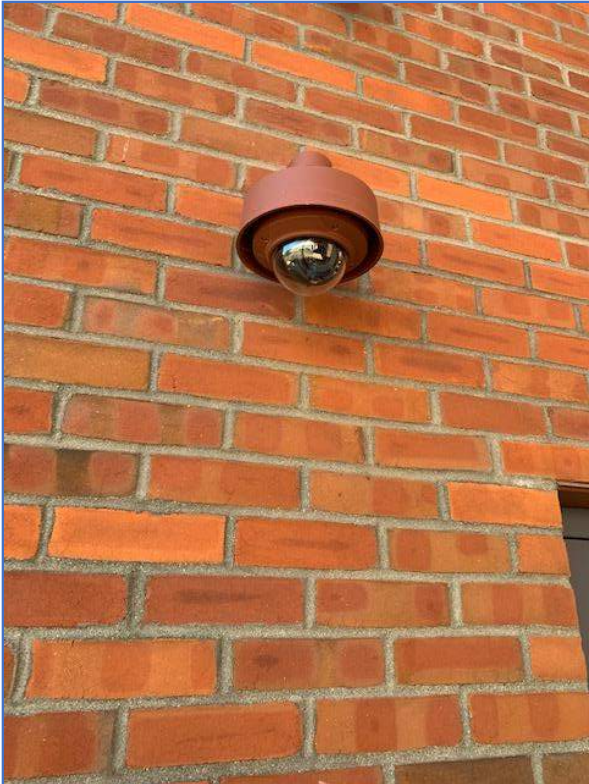
Security System Photo 24 – Exterior Wall Mounted 180 Degree Security Camera with Custom Painted Casing
