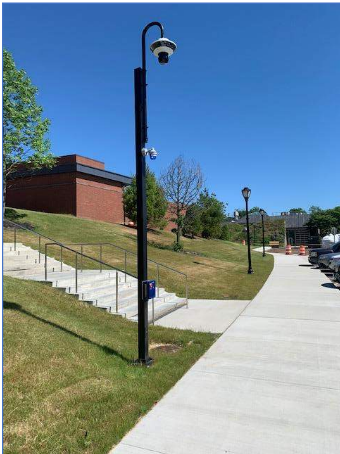
Security System Photo 23 – Exterior Pole with Emergency Telephone, Blue Light Strobe, and 360 Degree PTZ Security Camera
