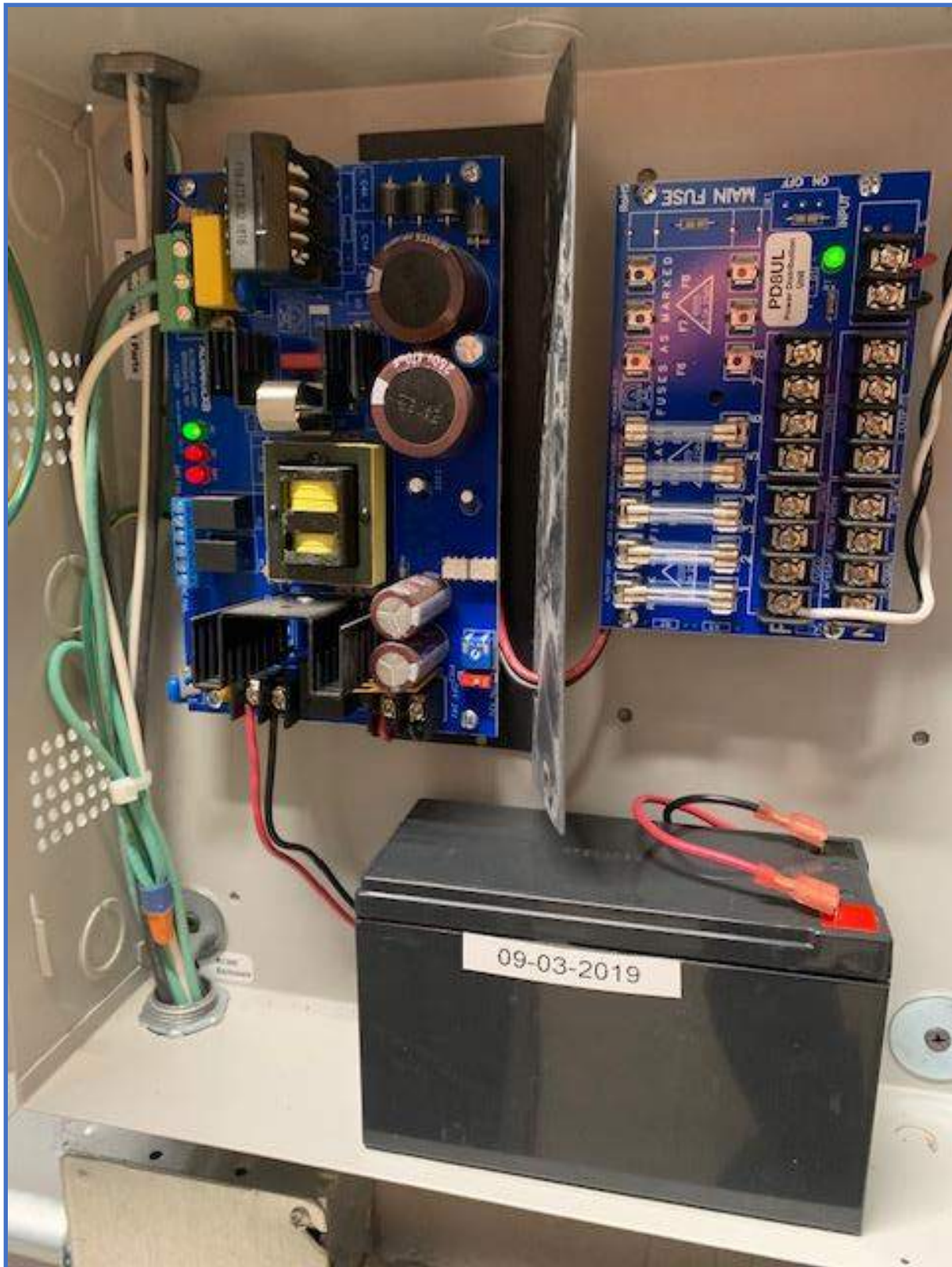
Security System Photo 8 – Access Control System Power Supply
