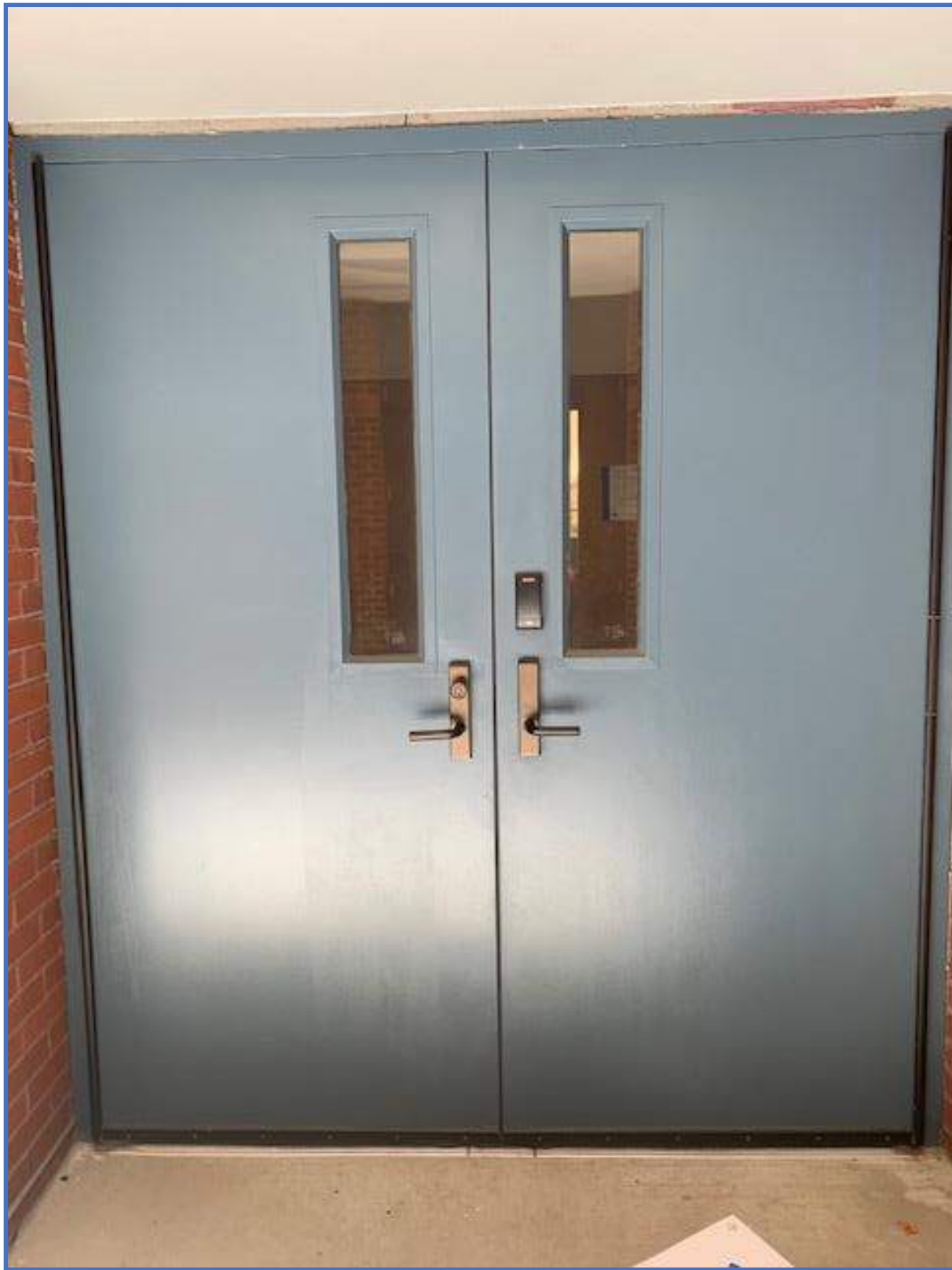
Security Systems Photo 3 – Access Controlled Double Door with Integrated Card Reader
