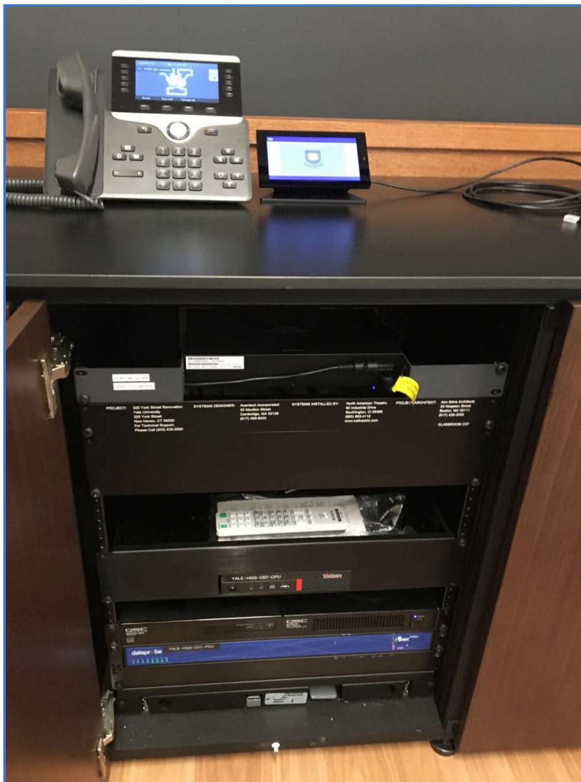
Conference Room Credenza Rack Photo 13 – Touchpanel Controlled QSC Q-Sys 1 Gbps AV over IP System with Local Room PC, Amplifier, IP Encoder/Decoder, Remote Controlled IP PDU
