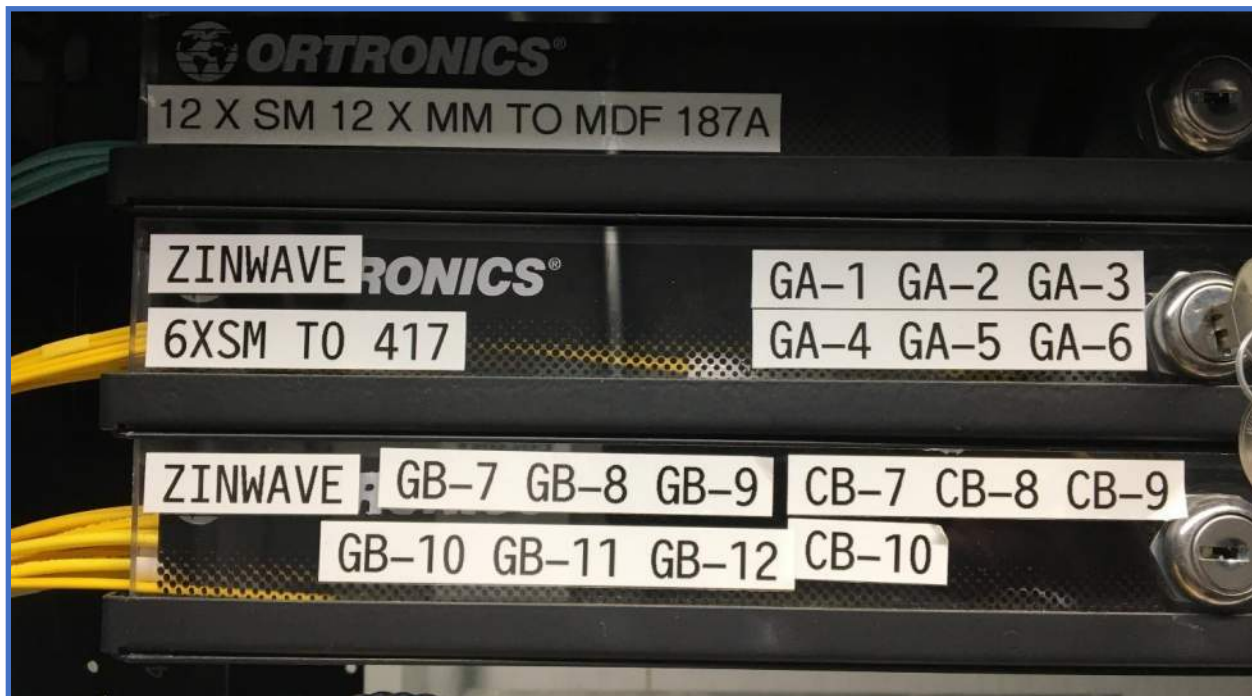
Distributed Antenna System Photo 33 – Singlemode Optical Fiber Termination Cabinet Labeling
