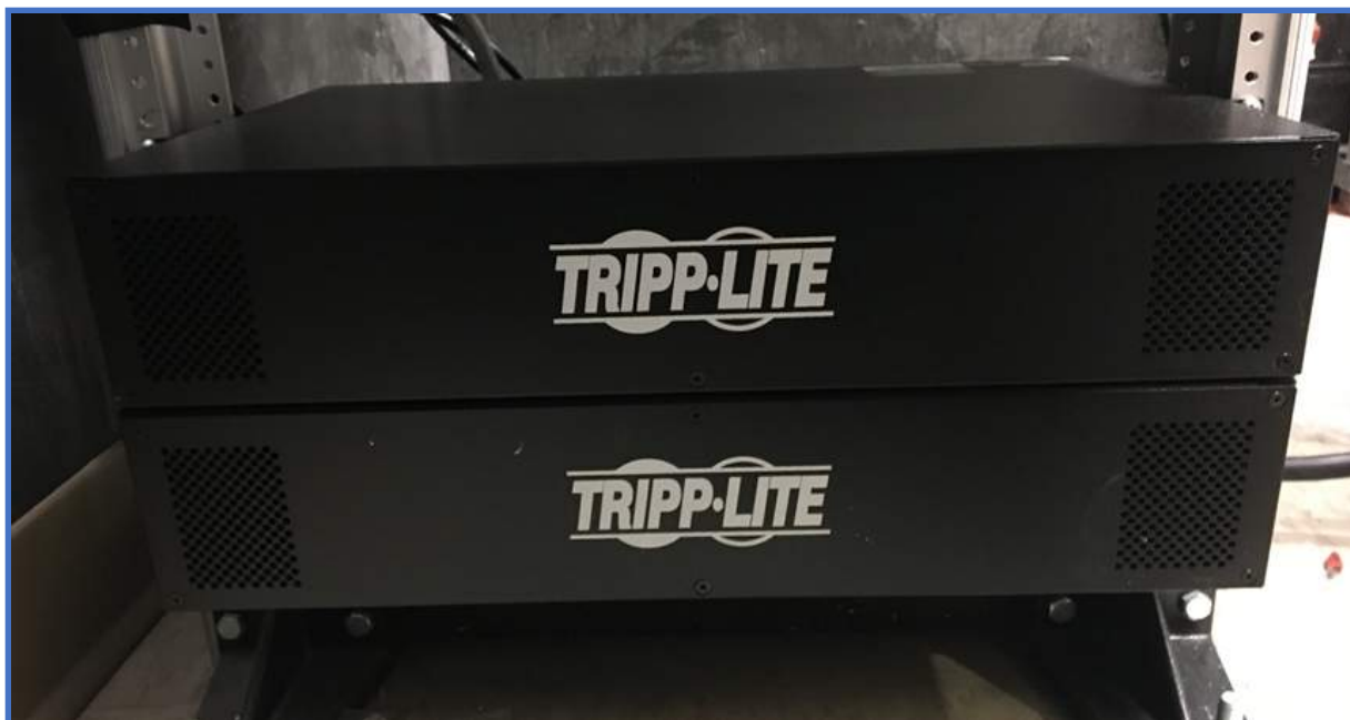
Network Electronics Photo 22 – Rack Mounted Redundant Power Distribution Units (PDU's)
