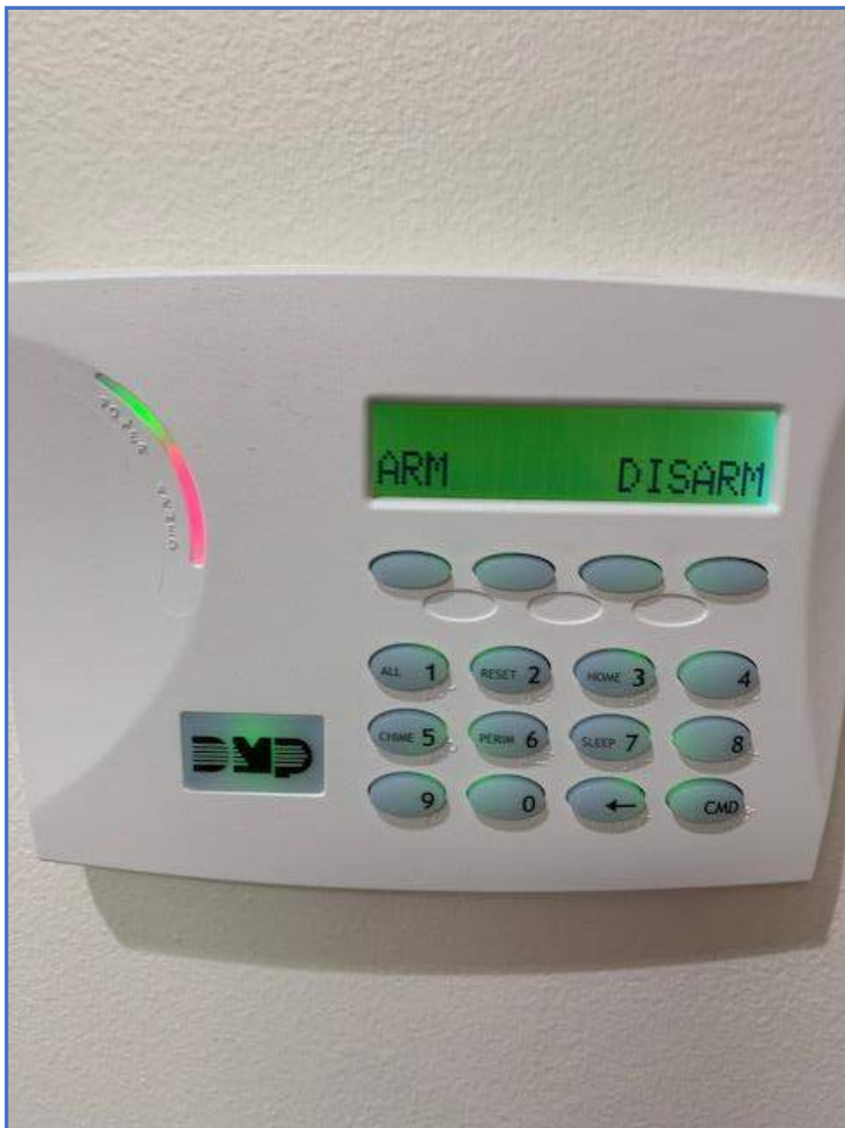
Security System Photo 12 – Intrusion Detection System Alarm Keypad
