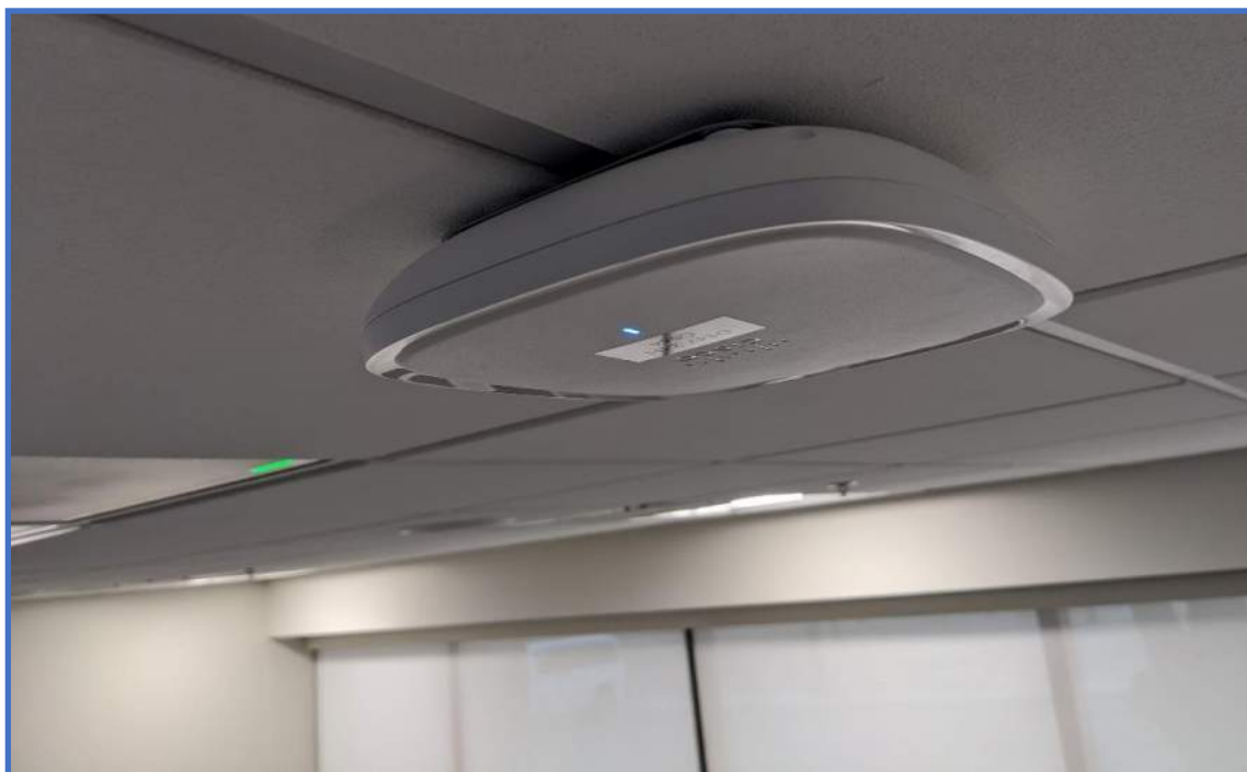
Wi-Fi Photo 36 – Ceiling Mounted Wireless Access Point
