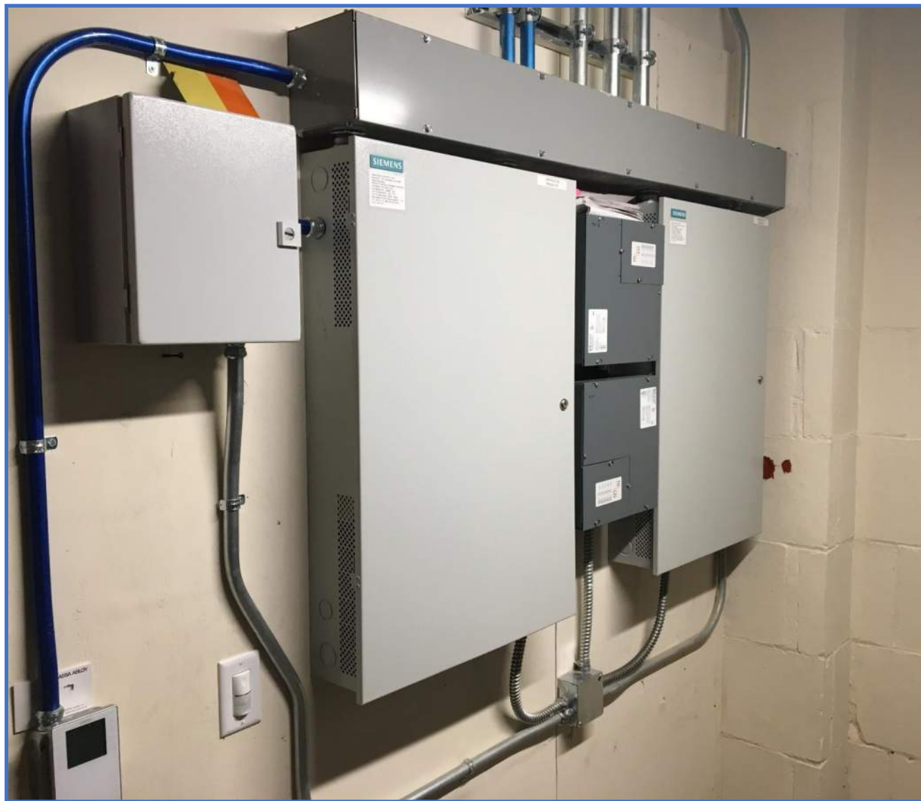
BAS Controls Headend Photo 44 – Building Controls System Headend Colocated in a Telecom Room
