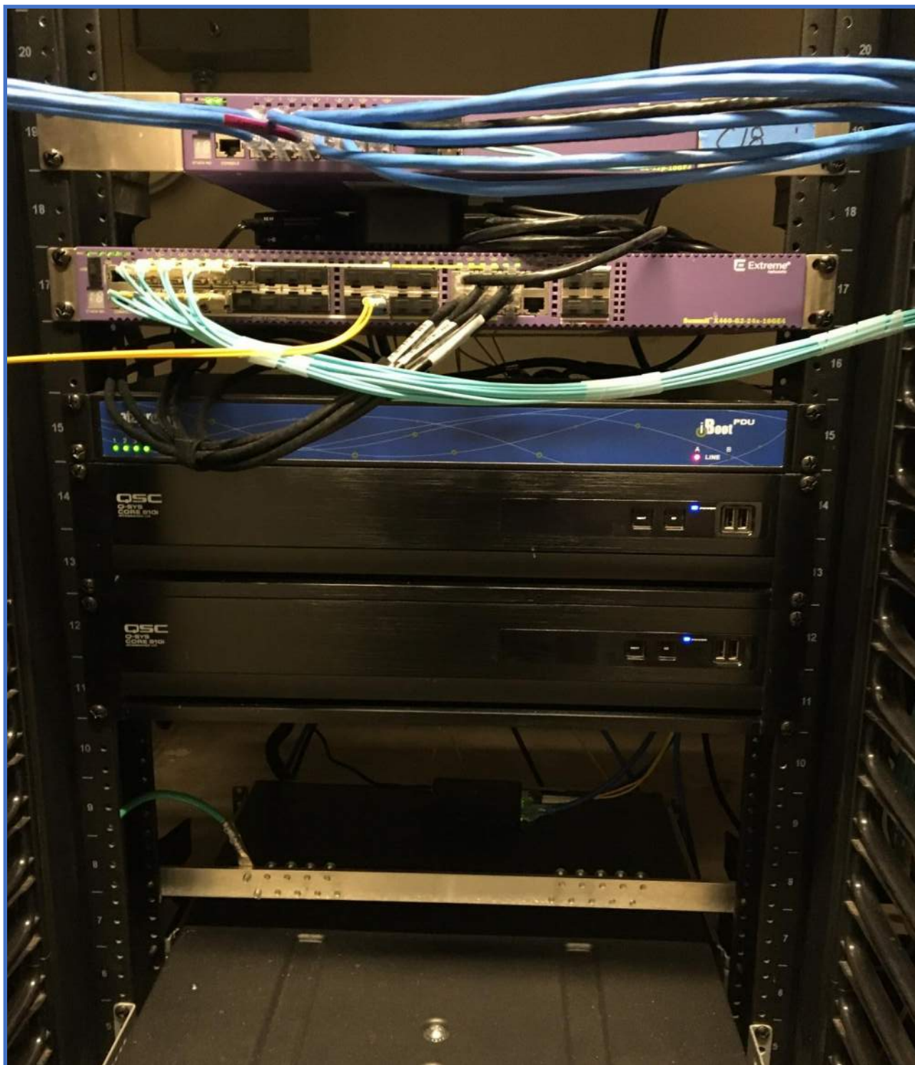
Telecom Room Audiovisual Equipment Photo 16 – Rack Mounted Audiovisual Equipment Headend for 1 Gbps AV over IP QSC Q-Sys System with Remote Redundant Core Processors and Remote Controlled IP PDU
