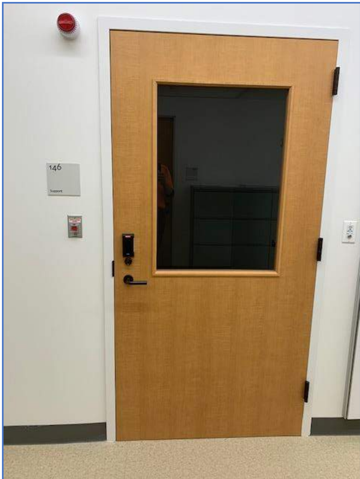
Security Systems Photo 2 – Access Controlled Single Door with Integrated Reader
