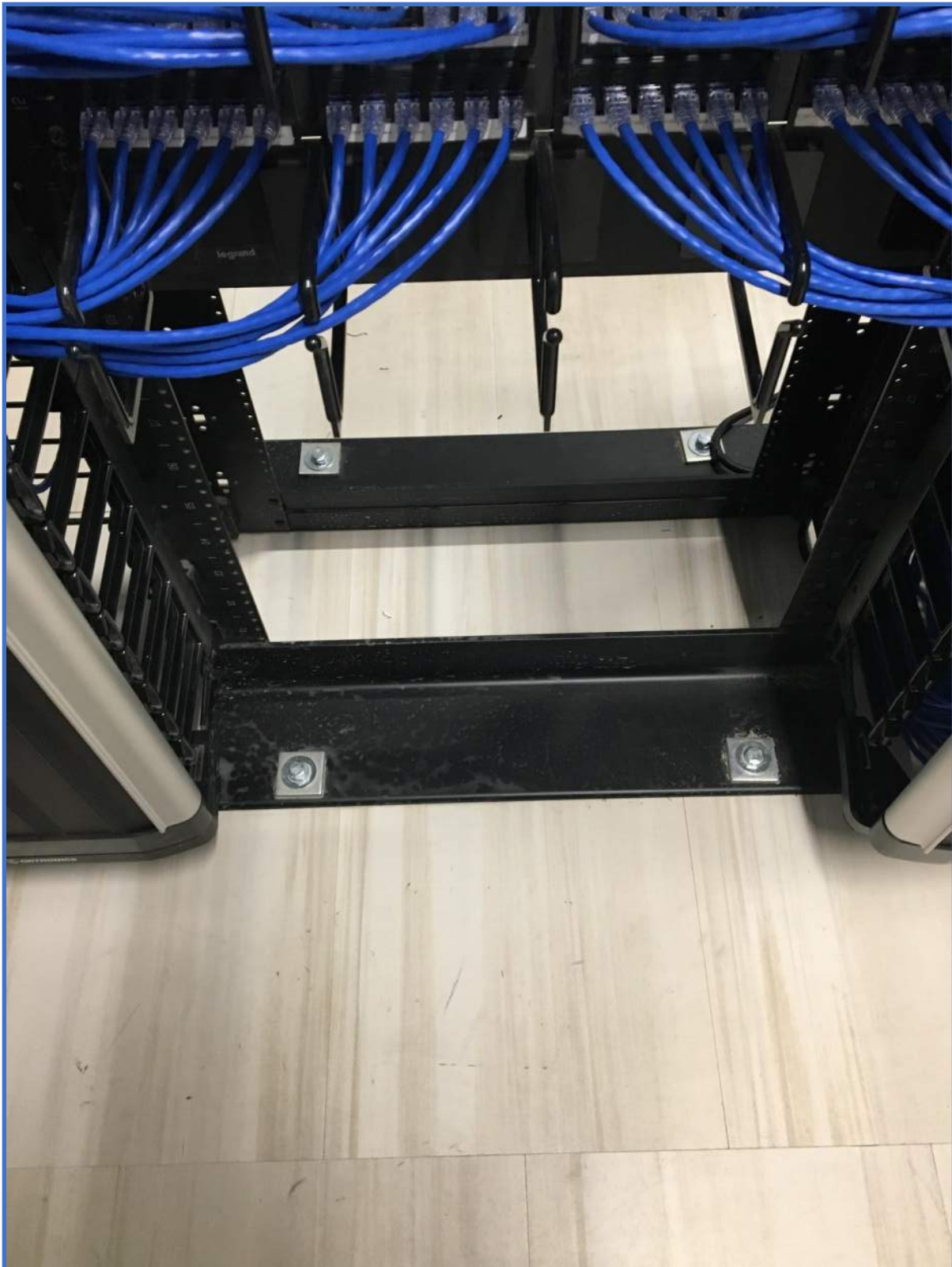
Cabling Equipment Rack Photo 17 – Equipment Rack Base Bolted to Floor
