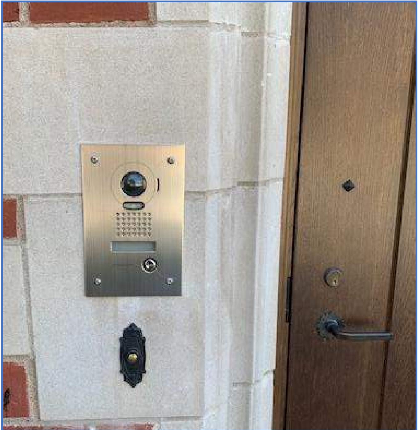
Security System Photo 17 – Video Intercom Substation at Exterior Entry Door
