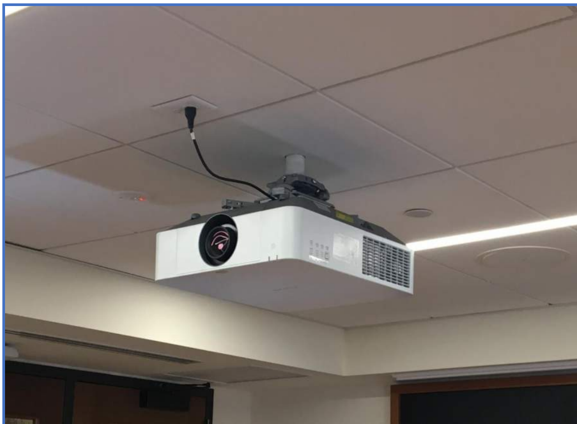
Ceiling Projector Photo 10 – Pendant Mounted Projector in Finished Accessible Ceiling
