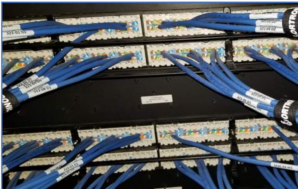
Incorrect Installation Photo 41 – RJ-45 Ports Shall Not Be Skipped in Patch Panel
