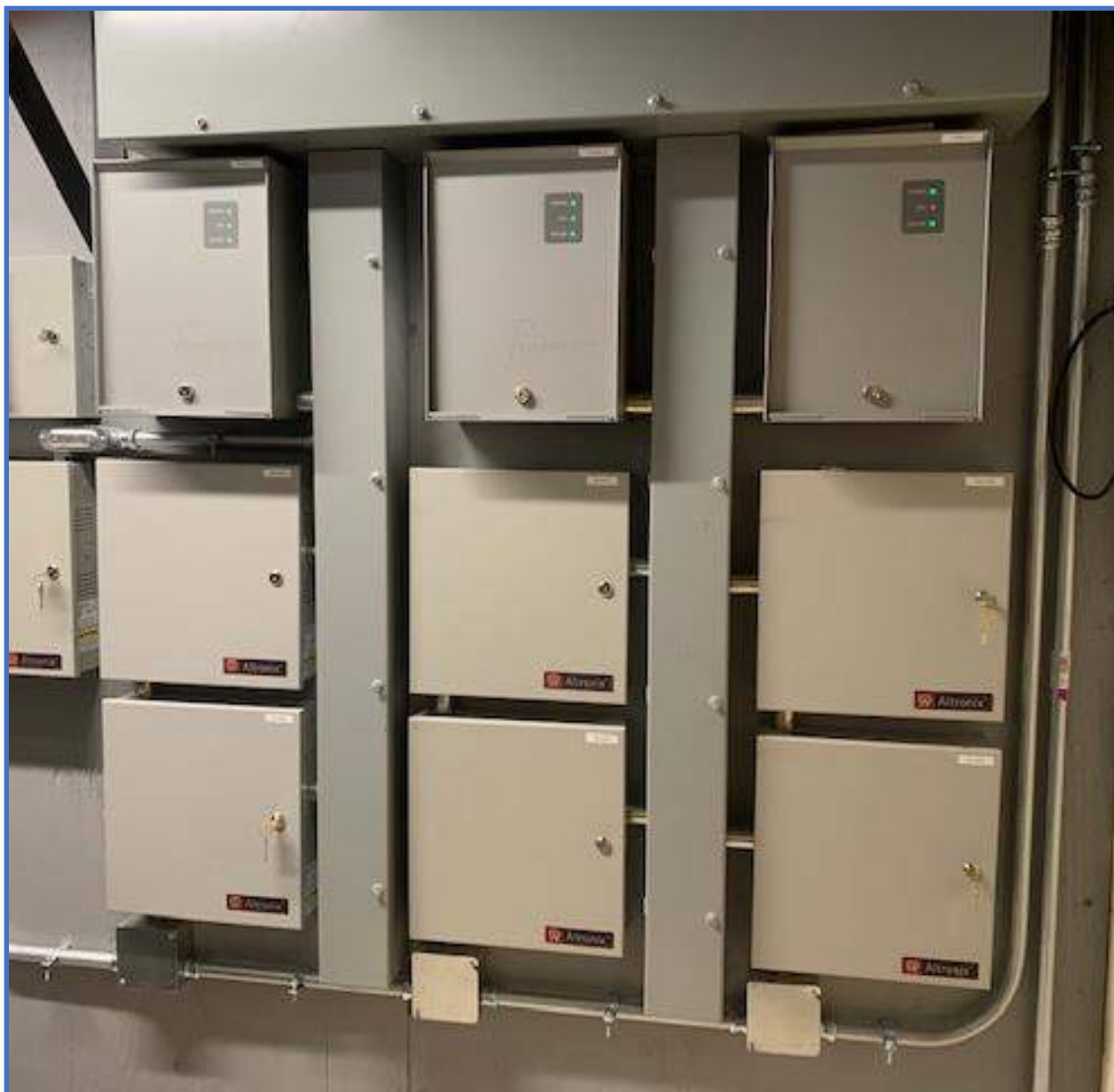
Security Systems Photo 6 – Access Control Panel Wallfield on Backboard in Telecom Room
