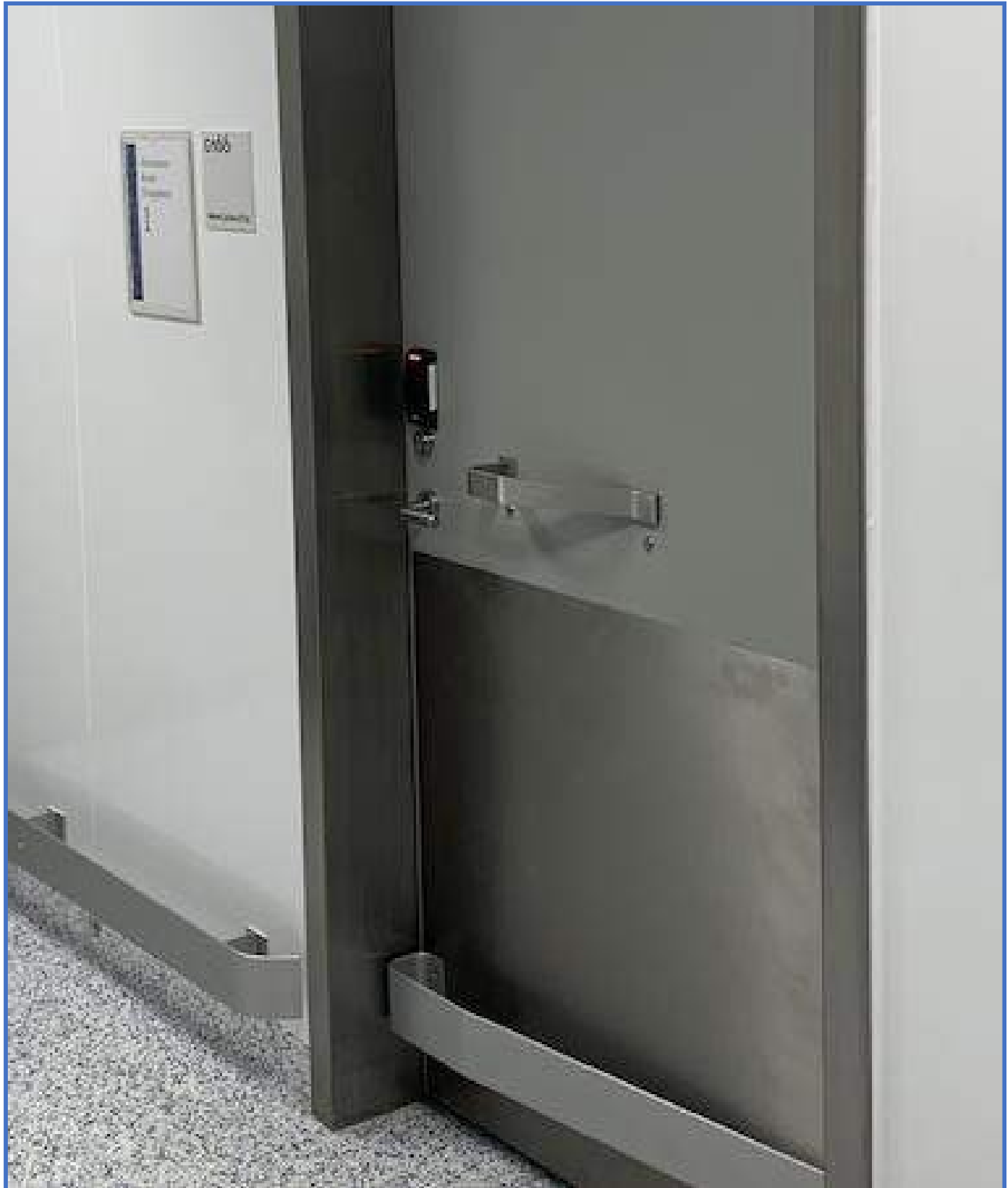
Security Systems Photo 5 – Access Controlled Vivarium Door
