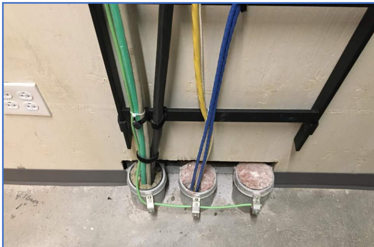
Telecom Outlet Photo 4 – Two (2) Category 6/Two (2) Strand 50 Micron OM4 with LC Duplex Connector for Fiber to the Desktop (FTTD) outlet
