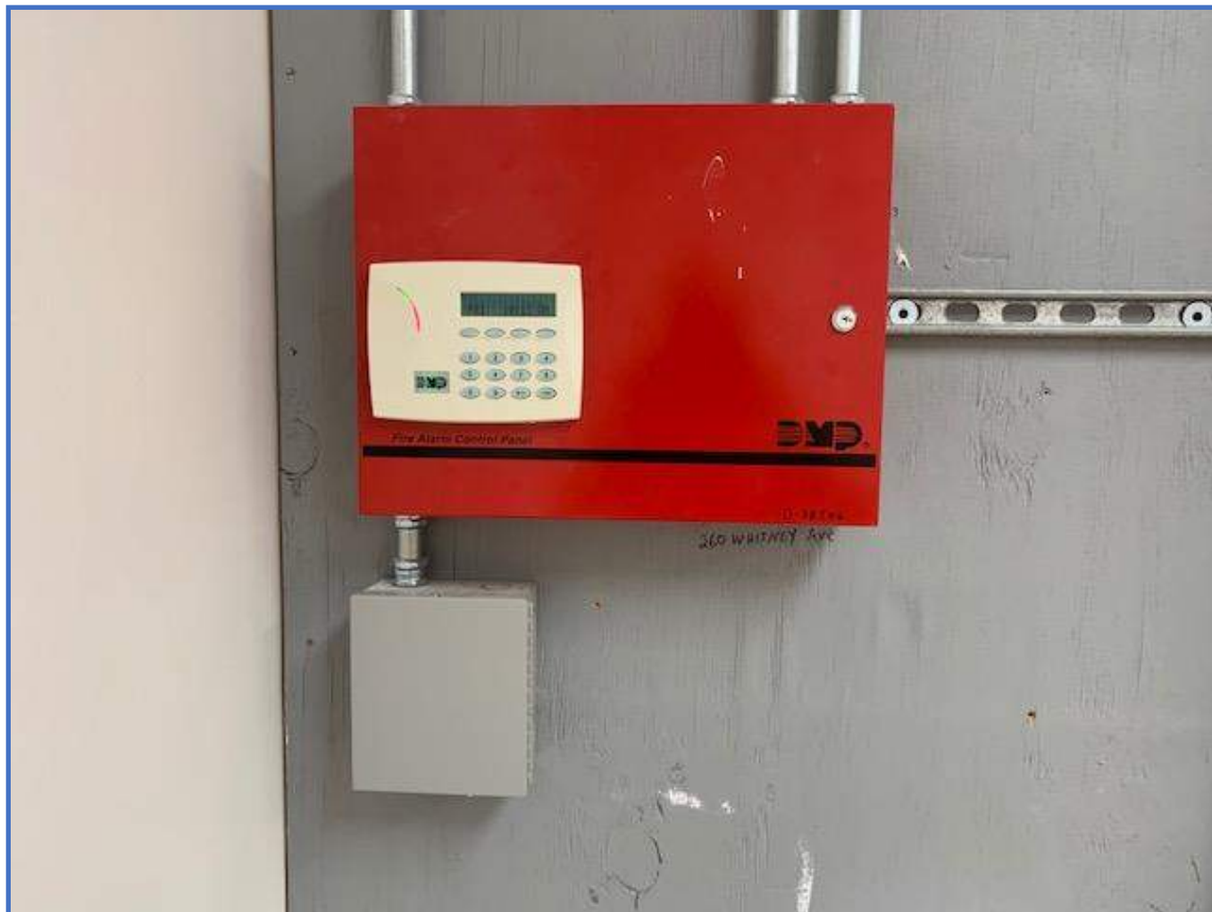
Security System Photo 11 – Alarm Panel (DMP) and Keypad Located at the Building Main Fire Alarm Panel for Central Station Communications
