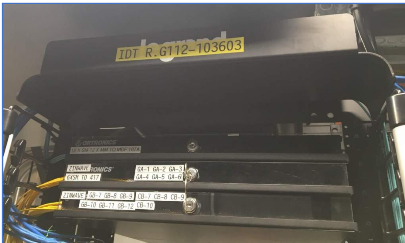
Distributed Antenna System Photo 31 – Singlemode Optical Fiber Termination Cabinet and Labeling
