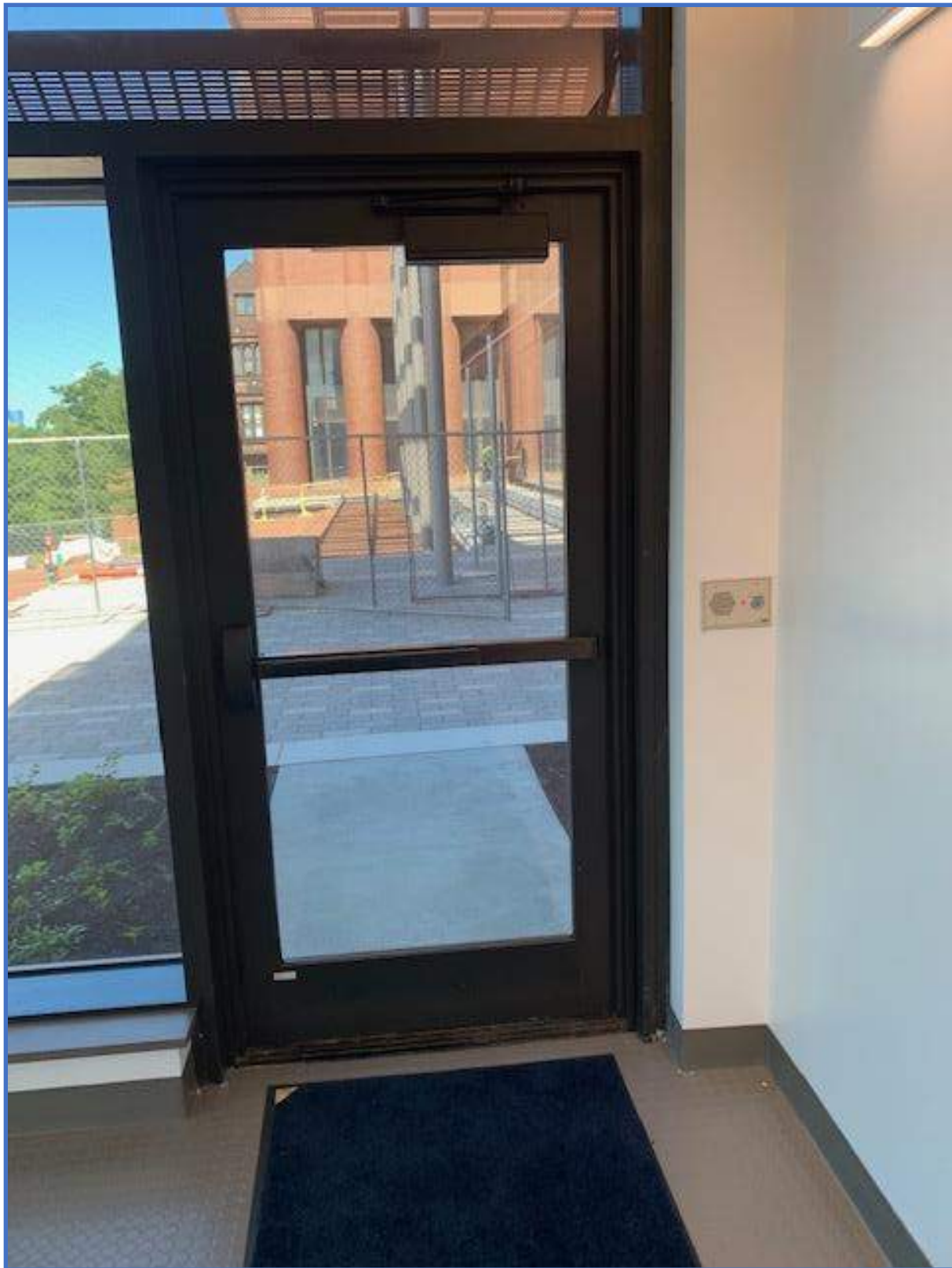
Security System Photo 14 – Emergency Exit Only Door with Door Management Alarm Panel
