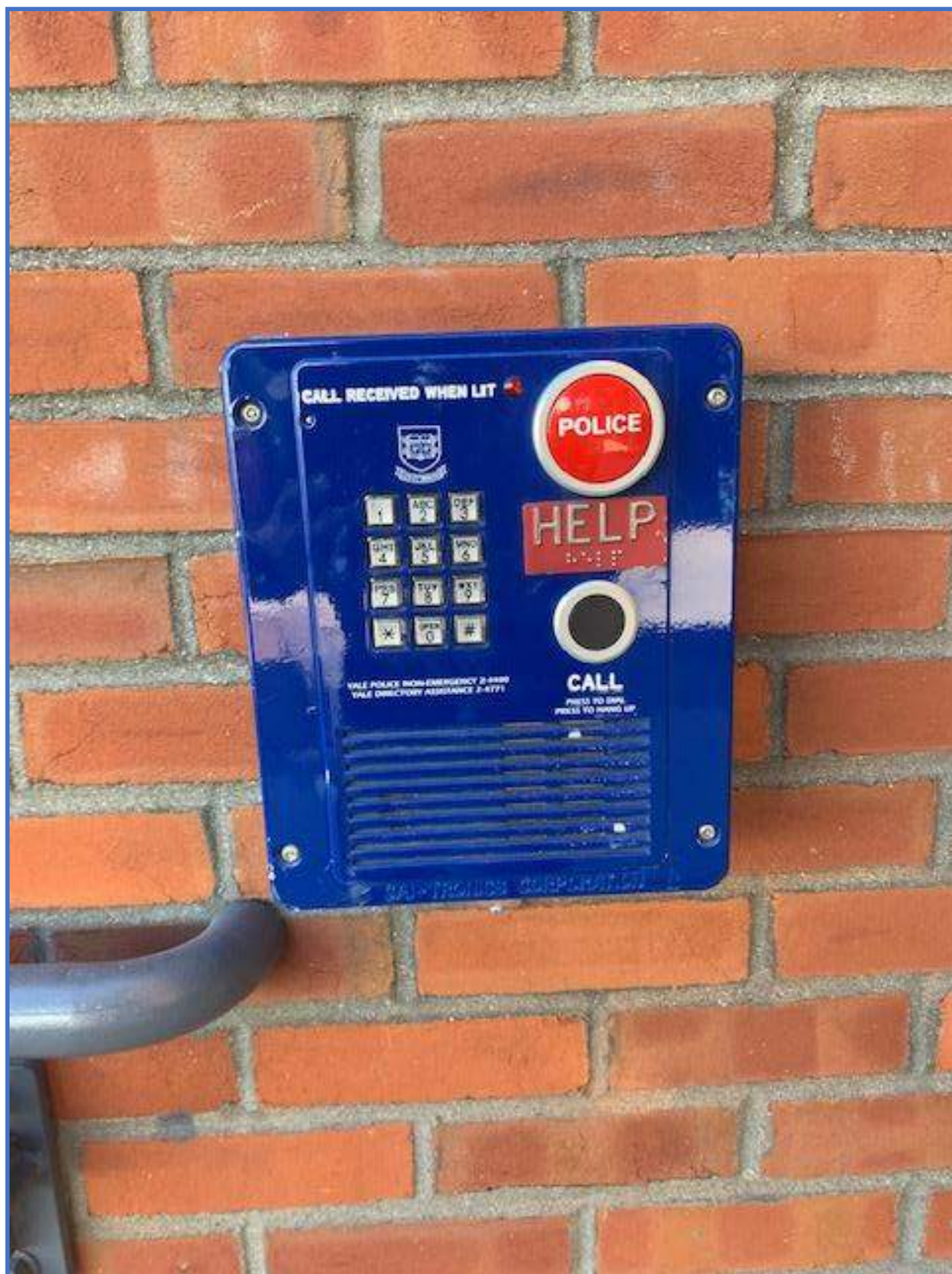
Security System Photo 19 – Exterior Emergency Telephone Call Station
