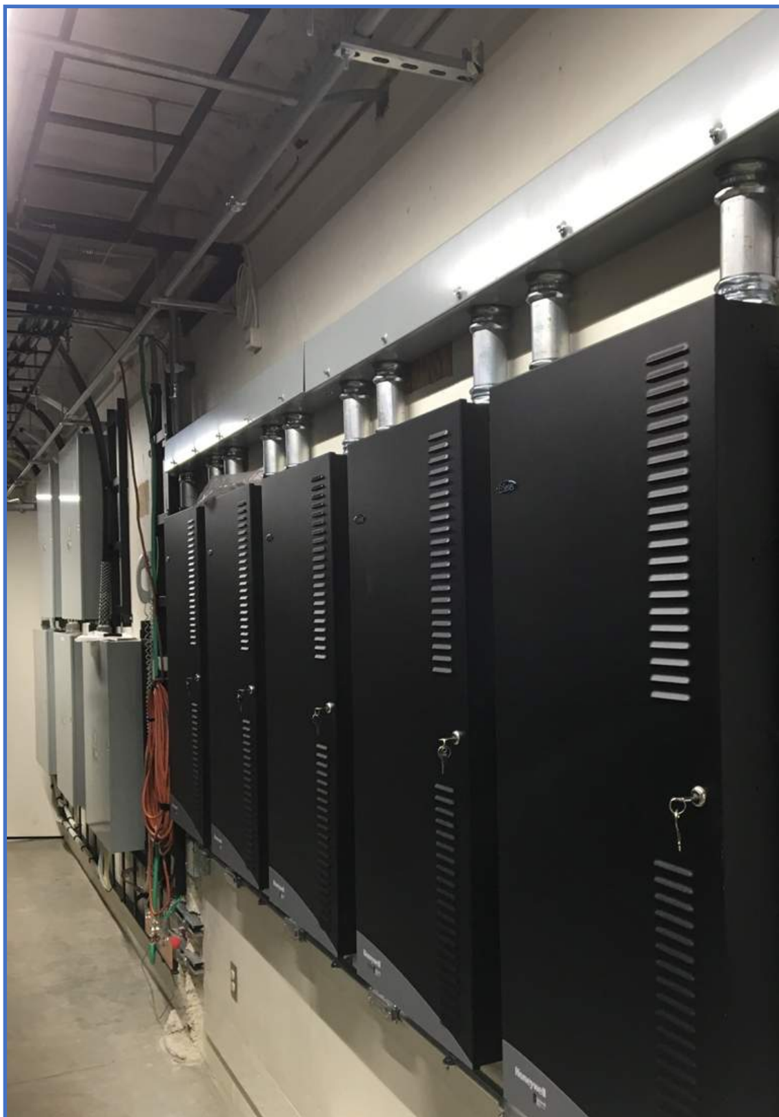
Fire Alarm Voice Evacuation (FAVE) System Photo 37 – FAVE Wallfield
