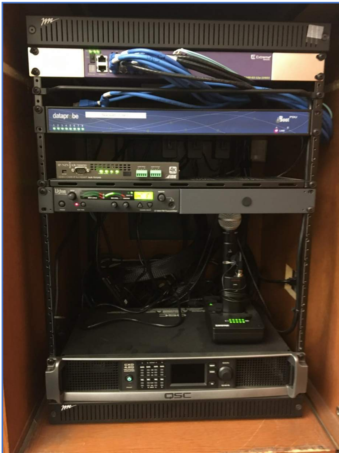
Audiovisual Cabinet Photo 1 - SDVoE 10 Gbps Audiovisual Cabinet Equipment Rack
