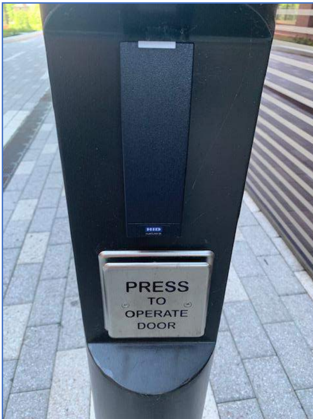
Security System Photo 16 – Exterior Entry Bollard with Card Reader, Automatic Door Push Pad Actuator
