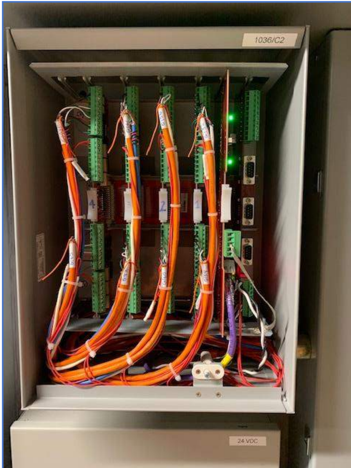
Security System Photo 7 – Access Control System Panel Terminations
