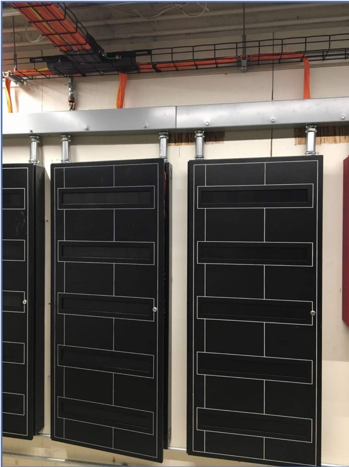
Fire Alarm Voice Evacuation (FAVE) System Photo 38 – Siemens FAVE Wallfield
