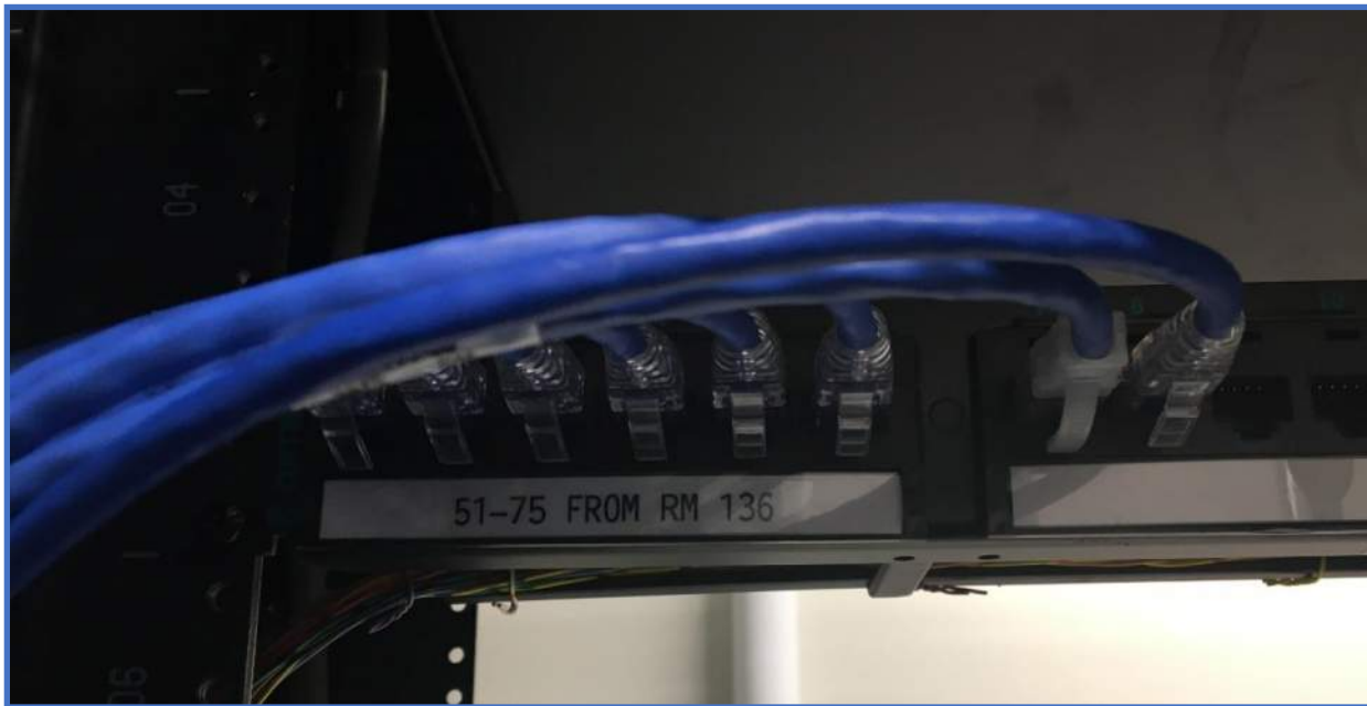
Labeling Photo 25 – Copper Voice Backbone Patch Panel
