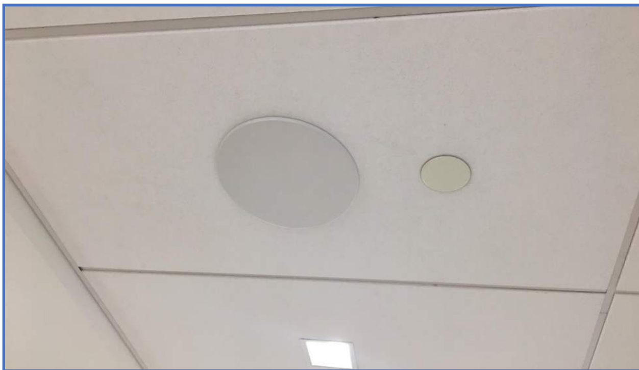
Distributed Antenna System Photo 34 – Ceiling Antenna
