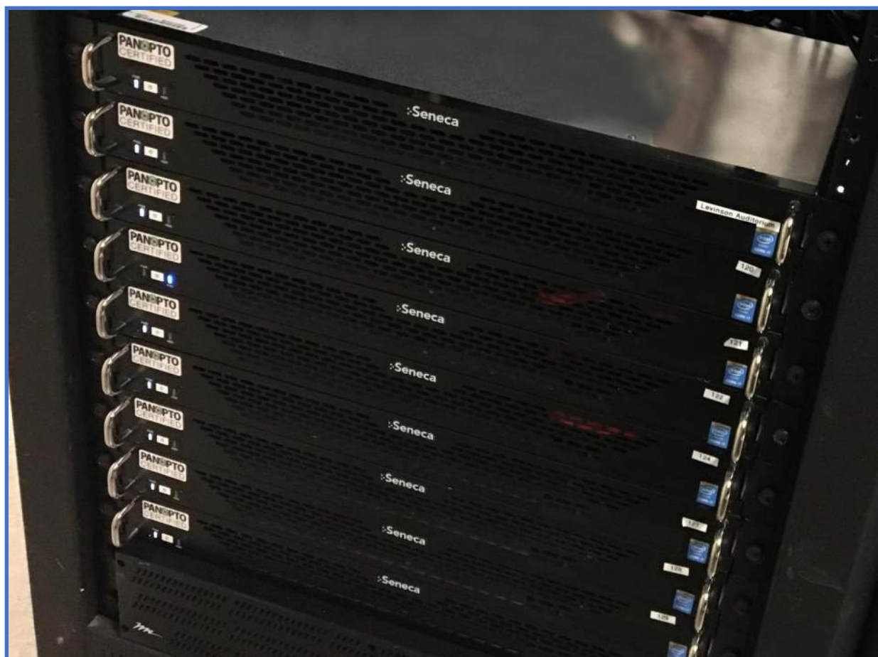
Audiovisual SDVoE Headend Photo 3 – Panopto-Certified Video Capture Appliances (by Seneca)
