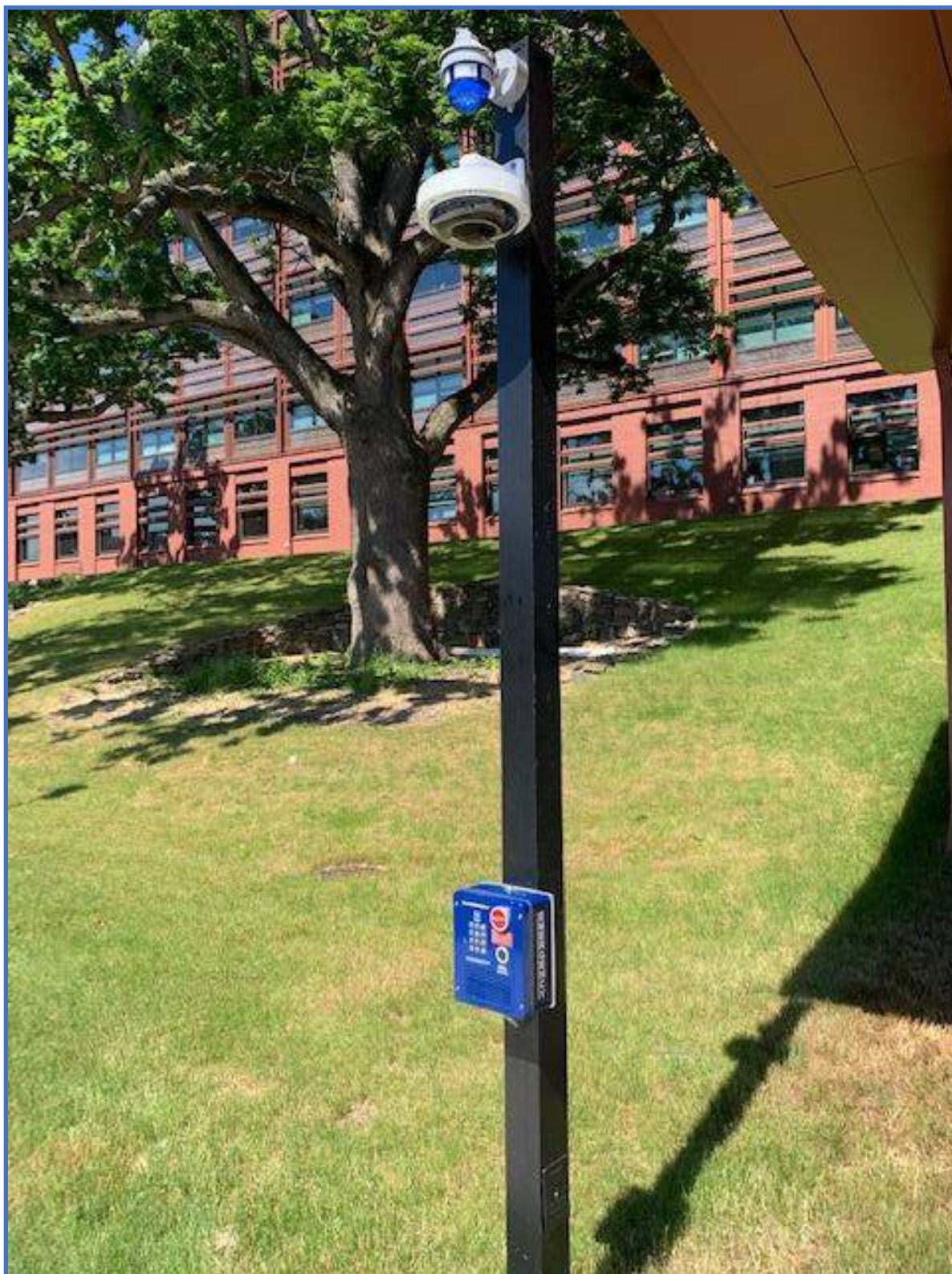
Access Control Photo 22 – Exterior Pole with Emergency Telephone, Blue Light Strobe, and Multi-Imager Security Camera
