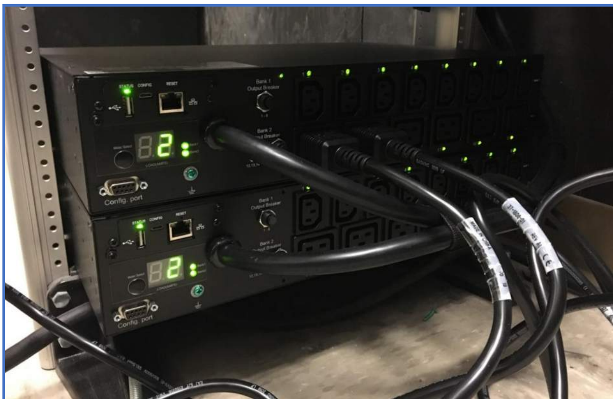
Network Electronics Photo 23 – Rack Mounted Redundant Power Distribution Units (PDU's)
