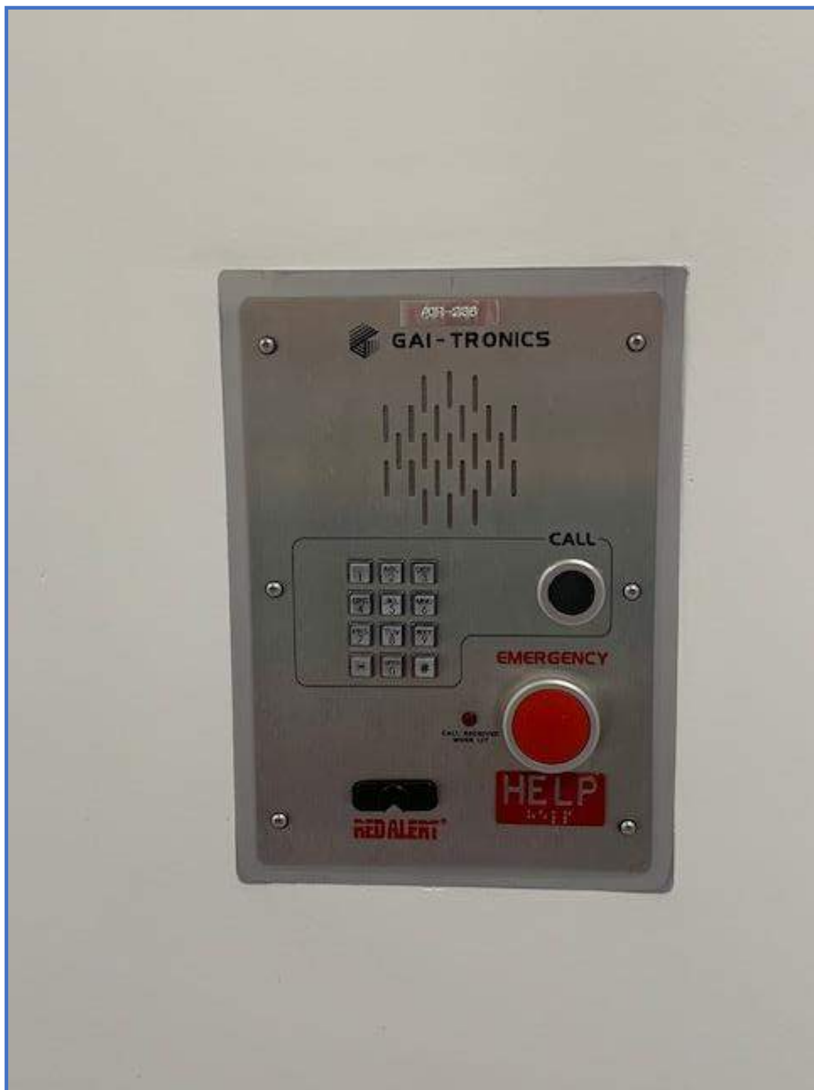
Security System Photo 18 – Interior Emergency Telephone Call Station
