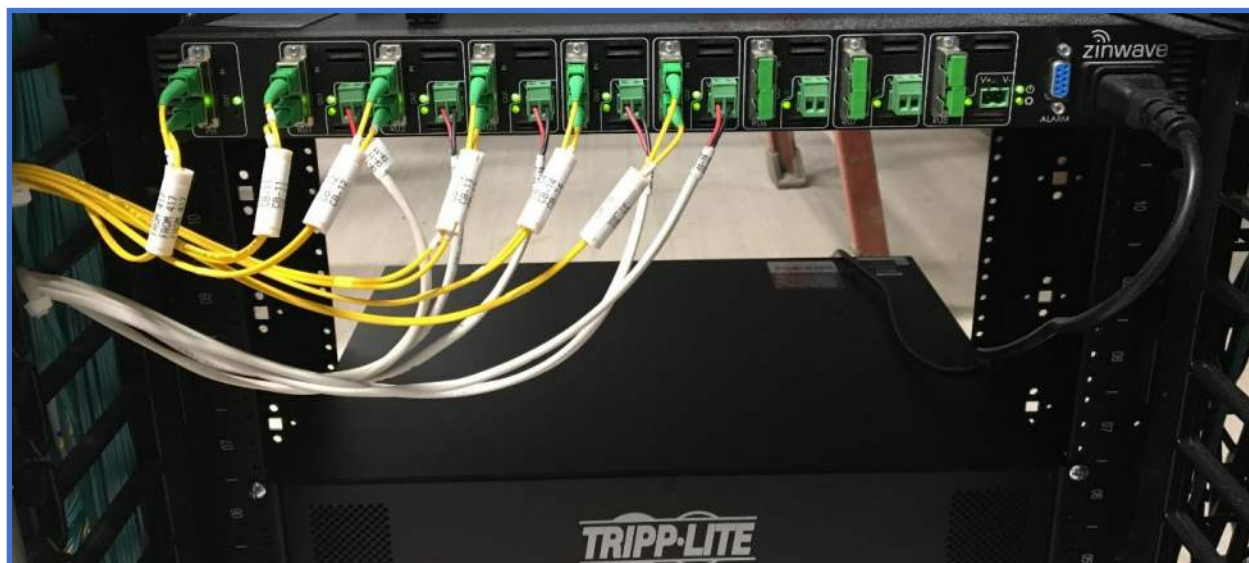
Distributed Antenna System Photo 32 – Optical Fiber and Low Voltage Hub Serving DAS Remote Units
