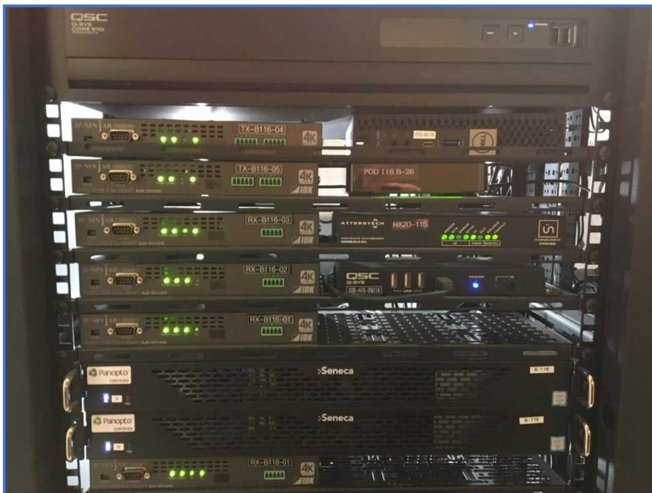
Audiovisual SDVoE Headend Photo 4 – Core Processor, Remote Classroom PC, Remote Wireless Presentation Device, SDVoE 10 Gbps OM4 Optical Fiber Extenders
