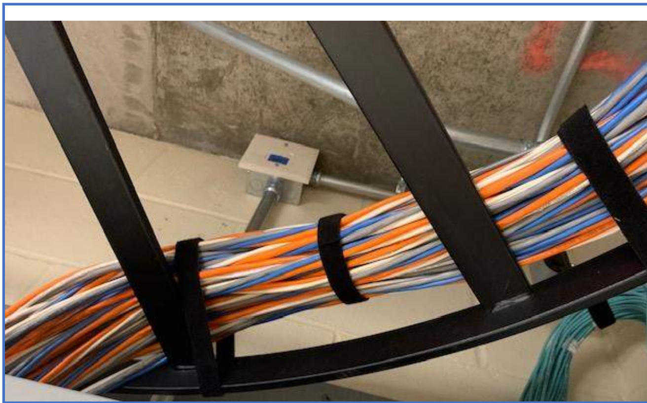
Security System Photo 10 – Access Control Composite Door Cabling Separated from Network Cabling within Telecom Room Cable Runways
