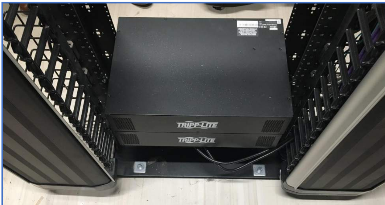
Network Electronics Photo 21 – Rack Mounted Redundant Power Distribution Units (PDU's)
