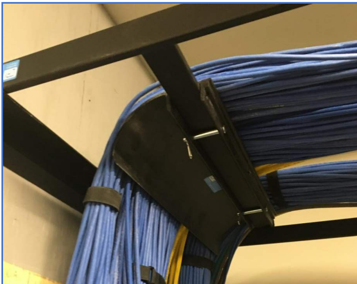
Telecom Room Cable Runway Photo 14 – Waterfall Cable Drop Out
