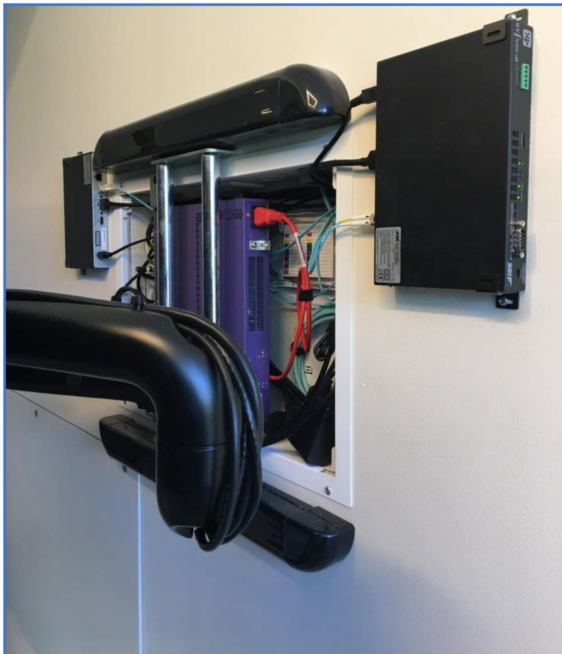
SDVoE 10 Gbps Flat Panel System Photo 12 - SDVoE 10 Gbps IP High Definition 4K Transmitter/Receiver and Network Switch Via OM4 50 Micron Multimode Optical Fiber (IDK NJR-01UHD, Extreme X440-G2-12p-10GE4)
