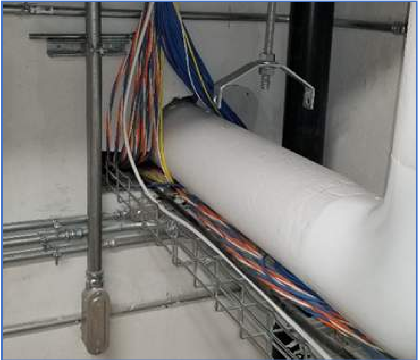
Incorrect Installation Photo 42 – Utility Routes Shall be Coordinated Unlike Depicted in this Photo
