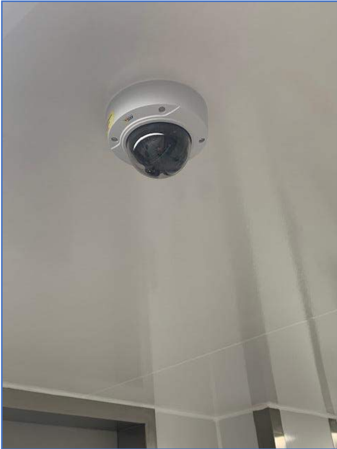
Security System Photo 25 – Ceiling Mounted Security Camera
