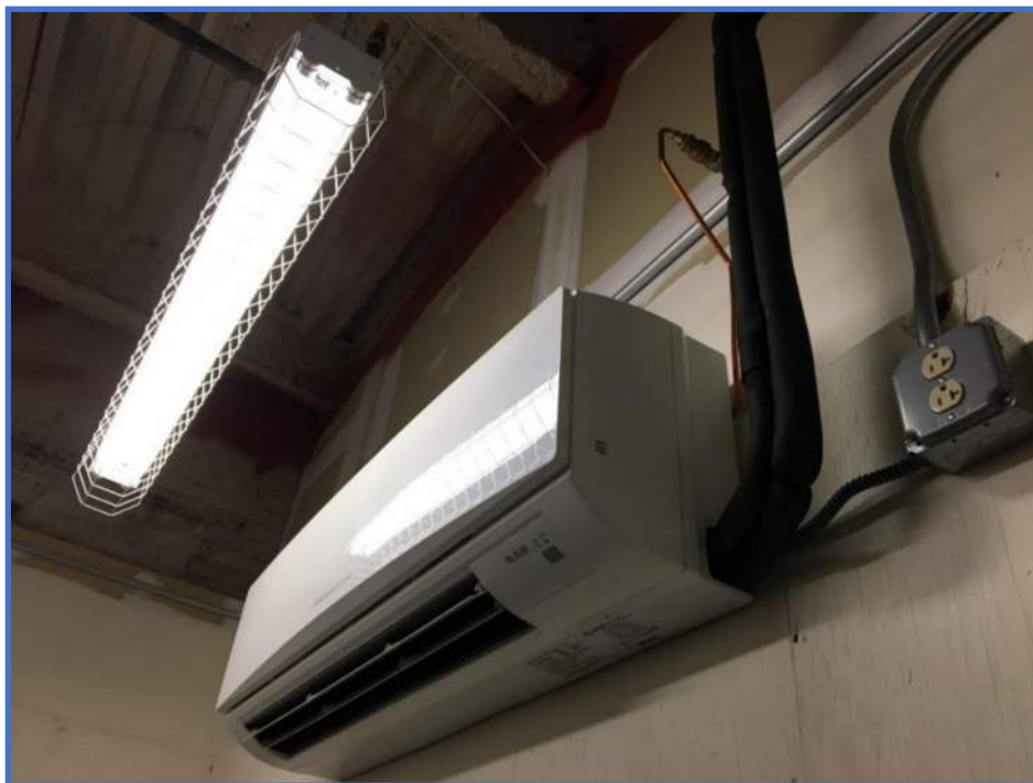
Telecom Room Photo 11 – Telecom Room Wall Mounted Evaporator Unit
