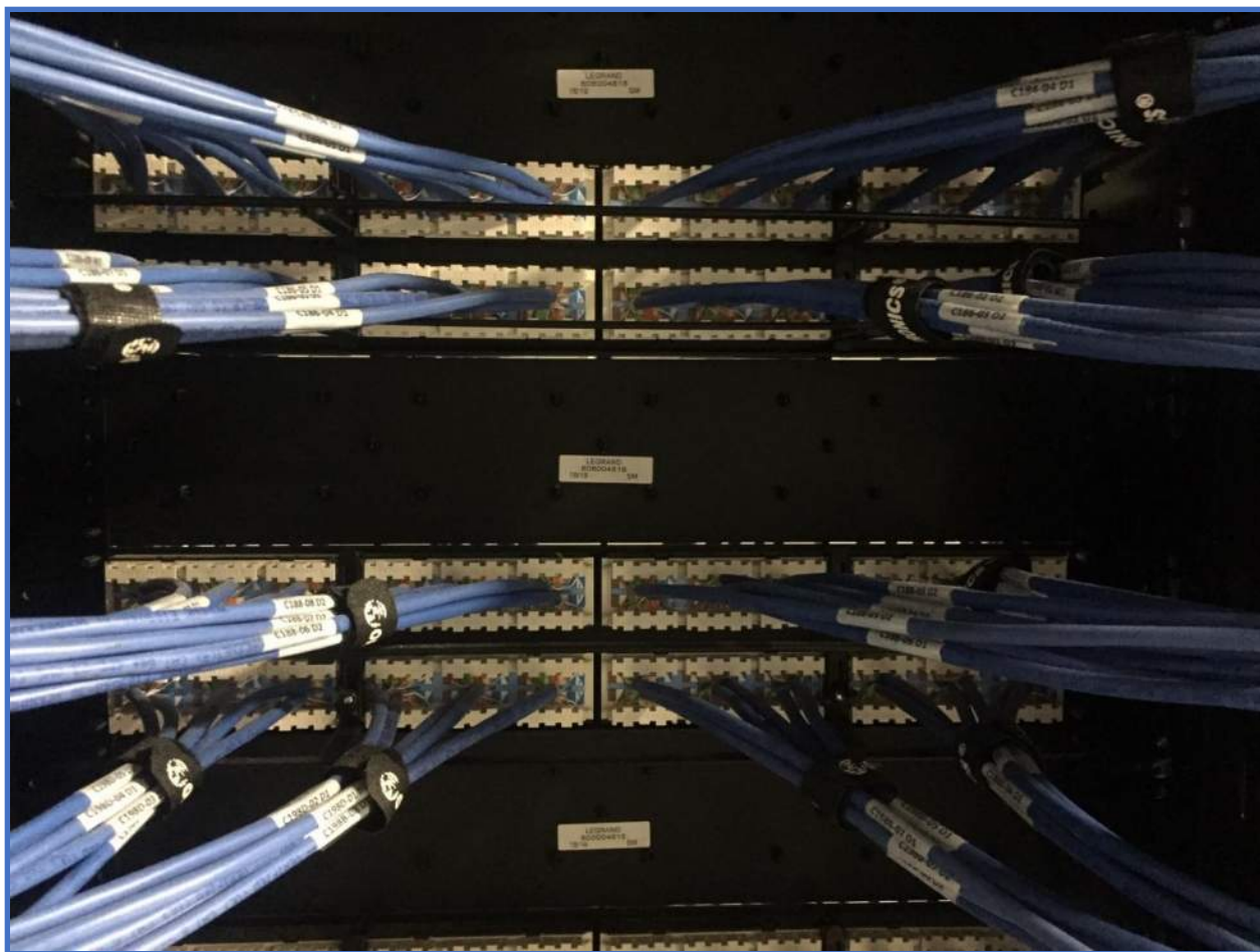
Cabling Equipment Rack Photo 18 – Patch Panel Cabling Termination, Labeling, Hook and Loop Fasteners, and Rear Cable Management Bars (Flat Patch Panels)
