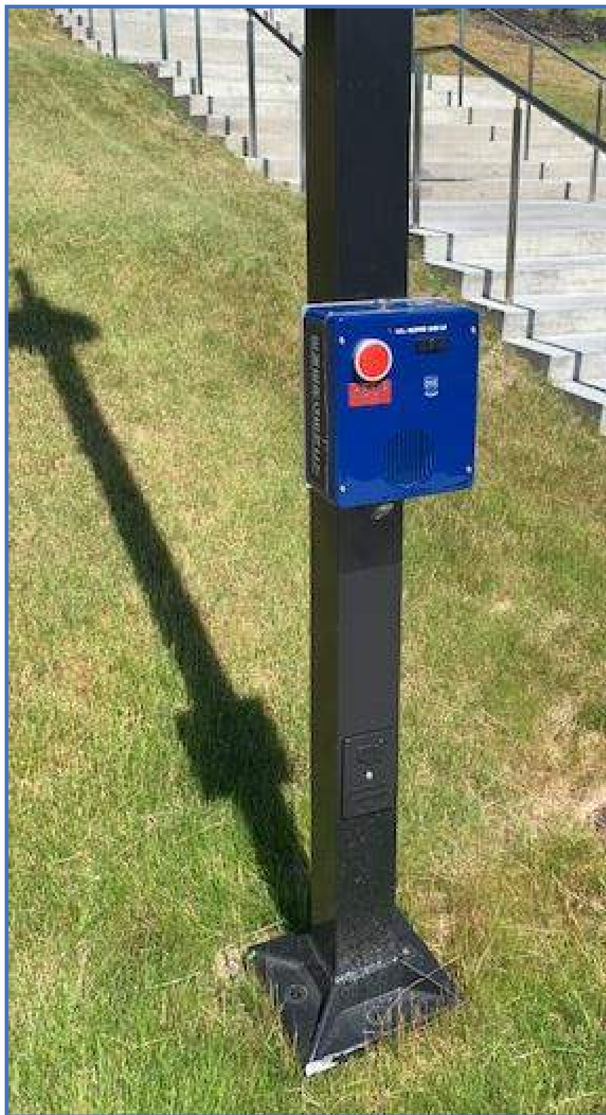
Security System Photo 21 – Exterior Pole Mounted Emergency Telephone
