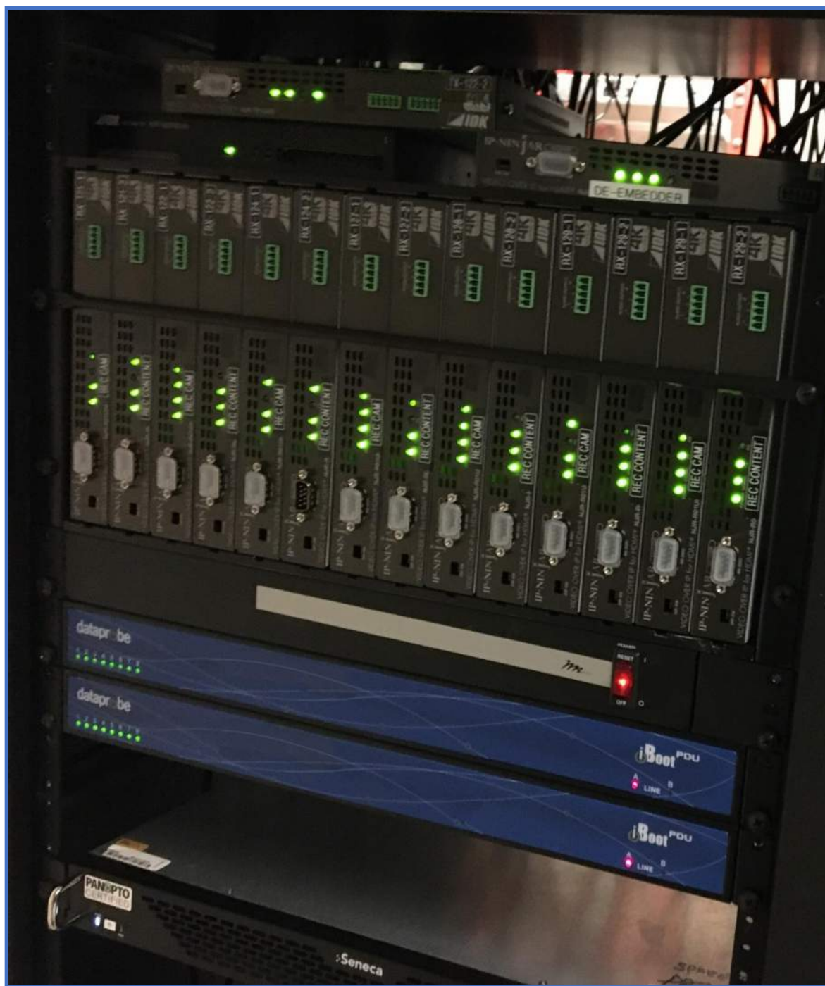
Audiovisual SDVoE Headend Photo 2 - SDVoE 10 Gbps IP High Definition 4K Signal Extenders Via OM4 50 Micron Multimode Optical Fiber
