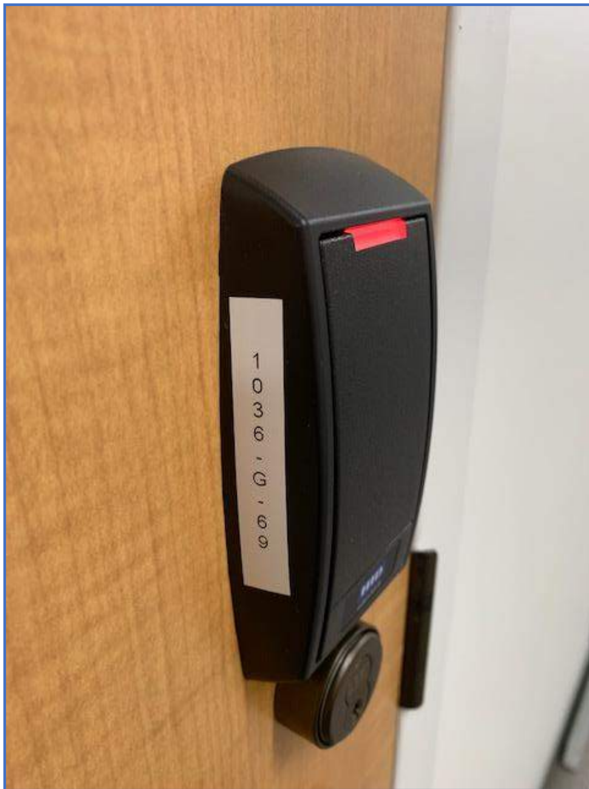
Security Systems Photo 1 – Labeled Integrated Mortise Card Reader with Door Position Switch and Request to Exit Switch
