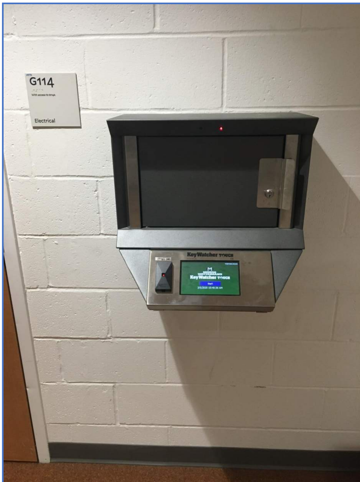
Security System Photo 26 – Morse Watchman Electronic Key Box
