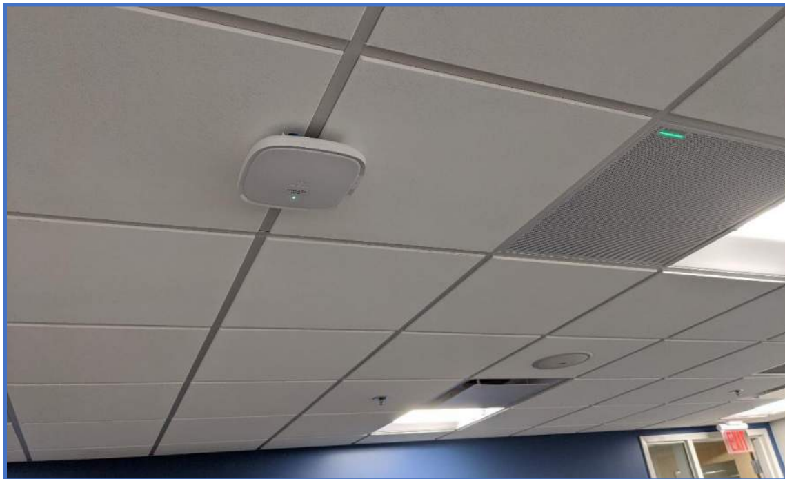
Wi-Fi Photo 35 – Ceiling Mounted Wireless Access Point
