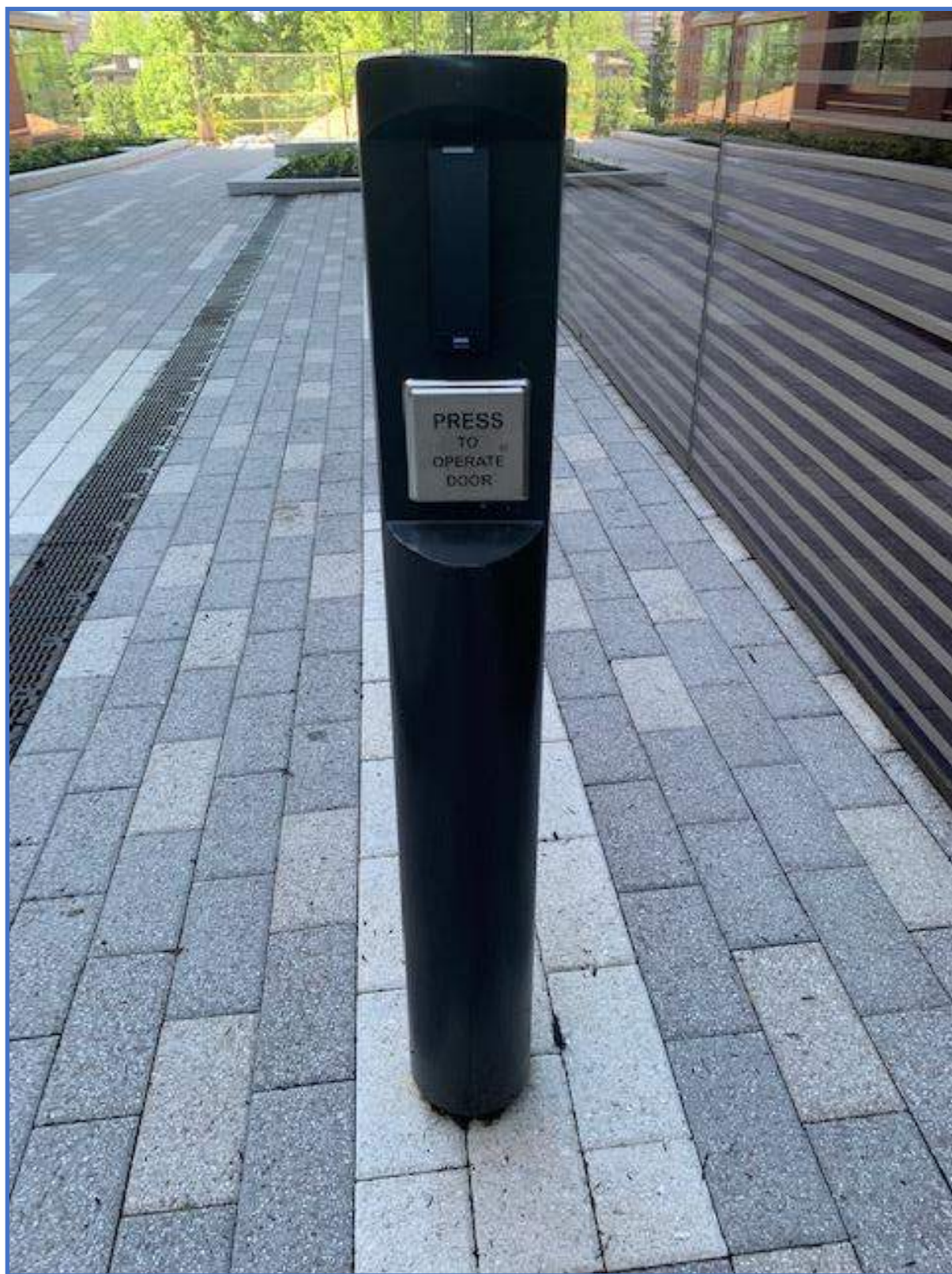
Security System Photo 15 – Exterior Entry Bollard with Card Reader, Automatic Door Push Pad Actuator
