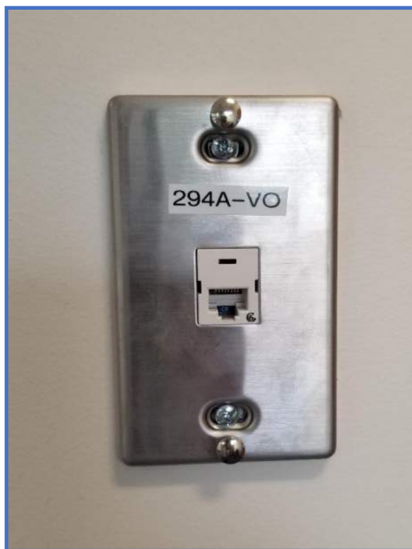
Telecom Outlet Photo 1 - Wall Mounted Telephone Outlet for Non-Cisco VoIP Telephone
