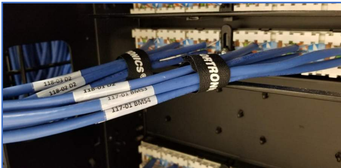
Cabling Equipment Rack Photo 15 – Back of Rack Cable Management
