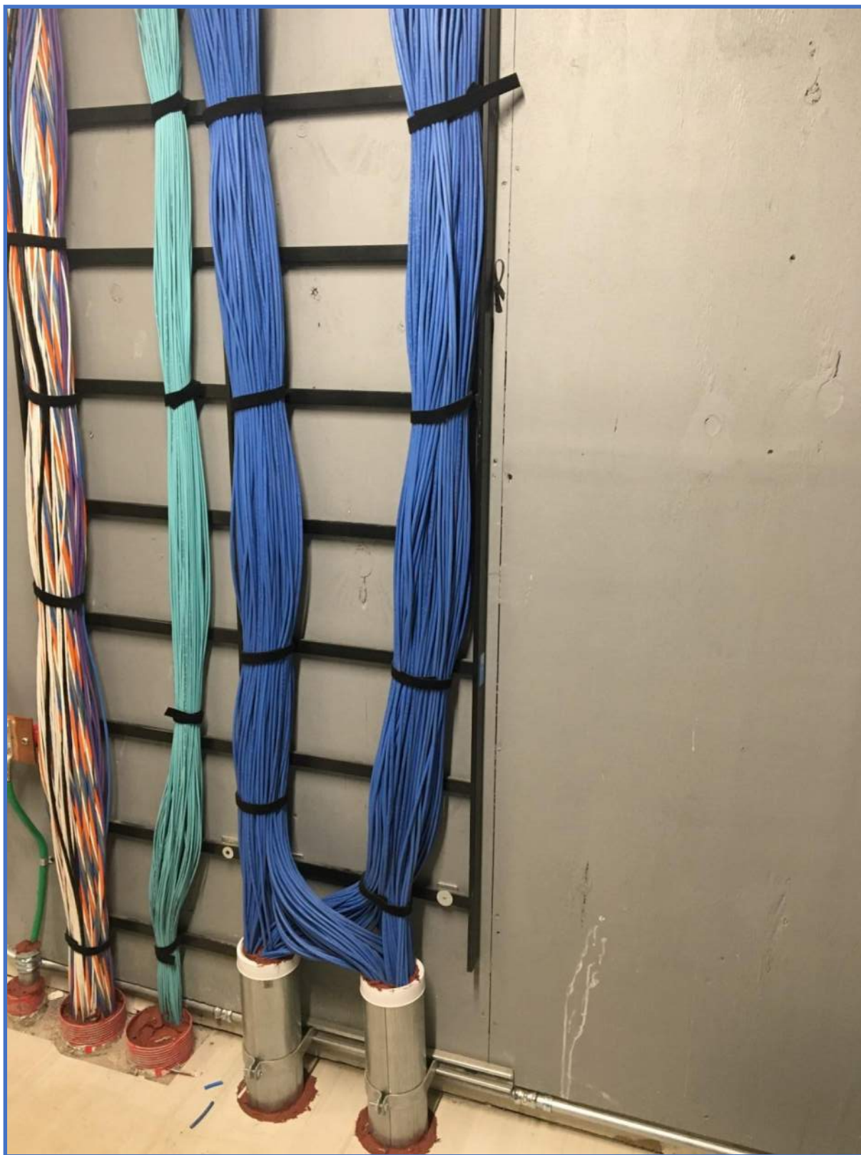
Telecom Room Cable Runway Photo 13 – Wall Mounted Vertical Cable Runway
