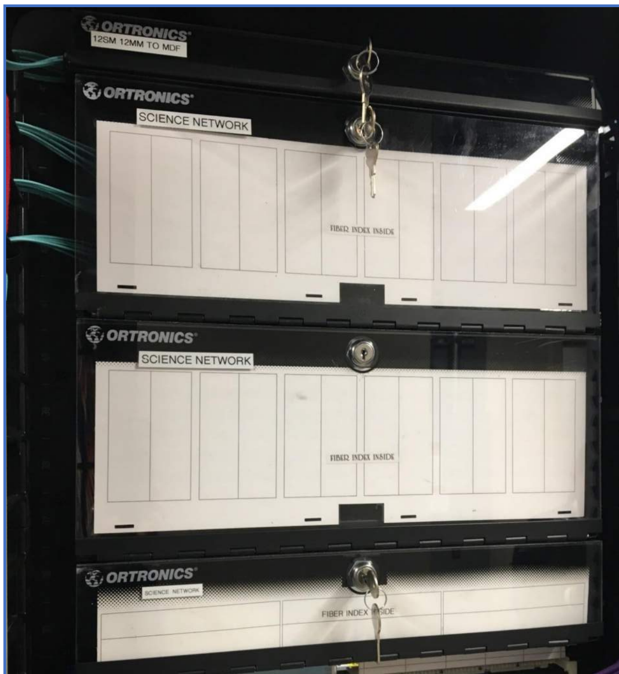
Science Network Photo 28 – OM4 50 Micron Multimode Science Network Optical Fiber Termination Cabinet
