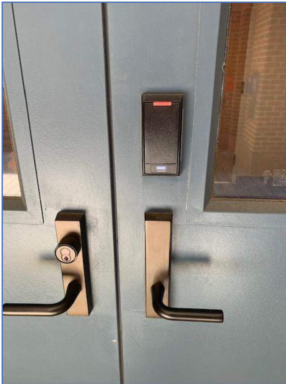
Security Systems Photo 4 – Integrated Card Reader, Right Hand Reverse Leaf of Double Door
